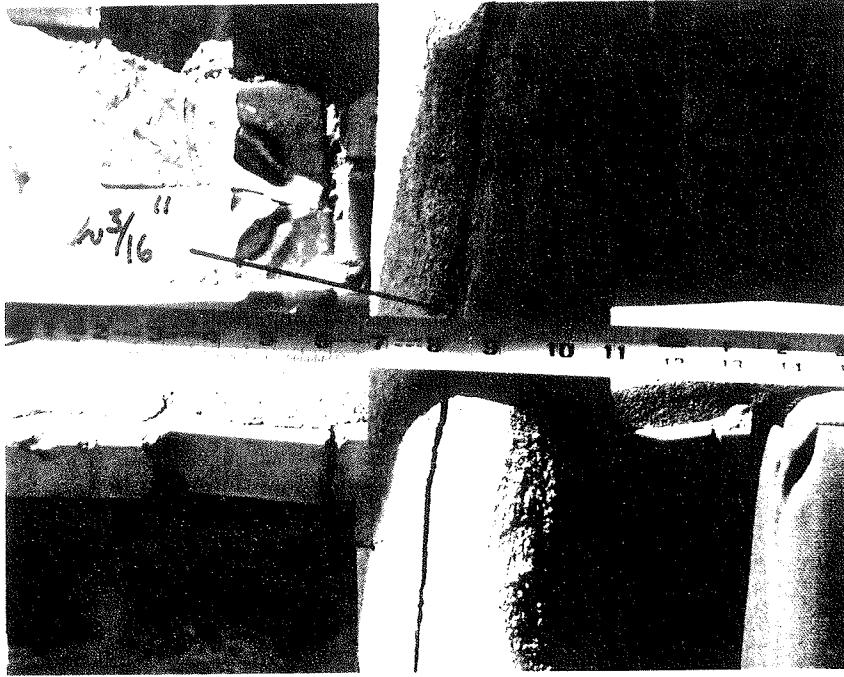
c) Indication of Existing Crack Gap
