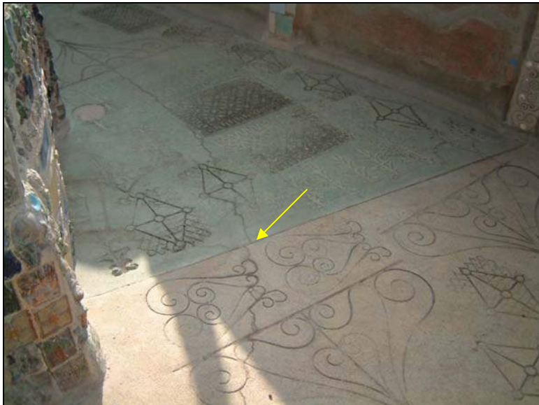
Photo 8. Crack bisecting section and crossing joint (arrow).
