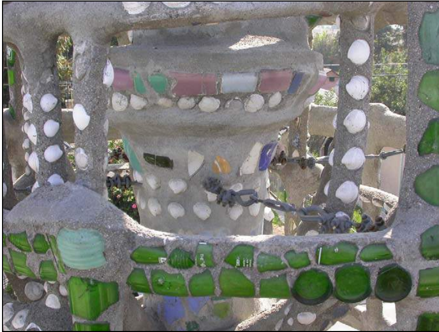
Figure 15: Cable bracing at Center Tower.
