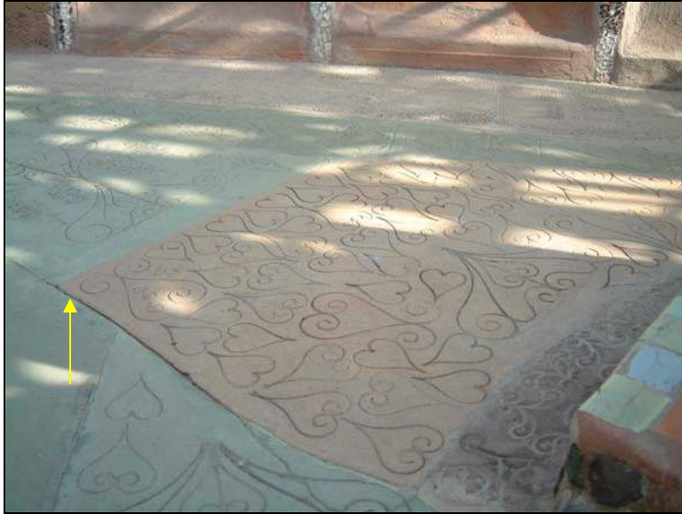
Photo 5. Slight uplift between colored sections just northwest of Center Tower (arrow).
