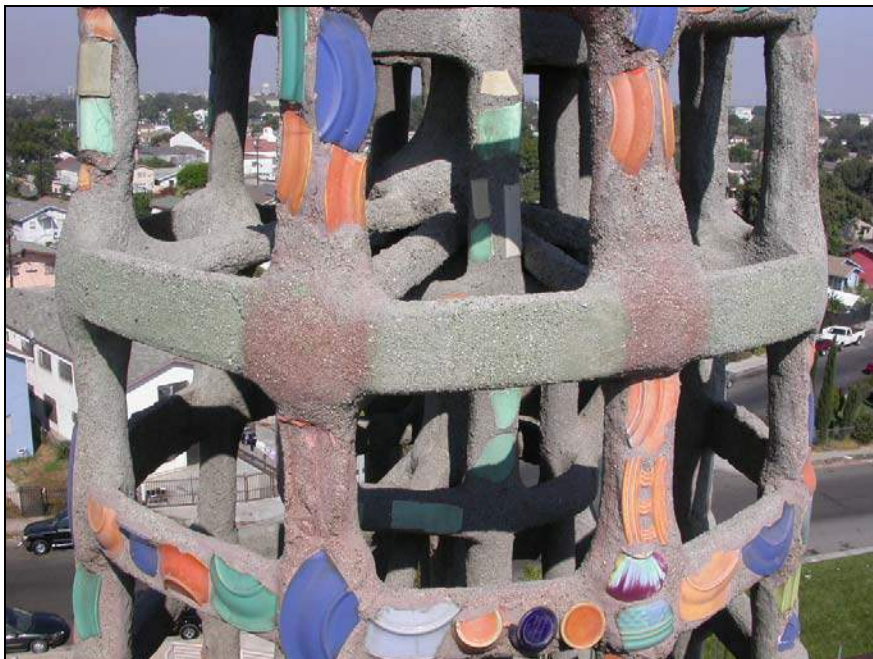
Figure 14: View of south elevation of Center Tower showing different mortar colors used.
