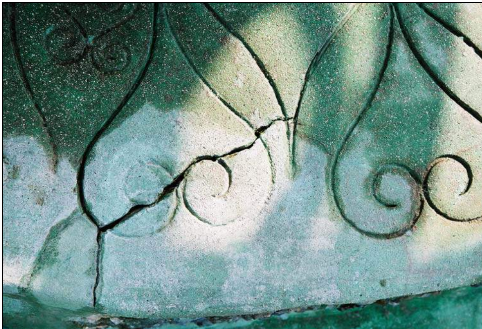
Figure 9: Mock-up no. 3 at west side of green base level of West Tower before treatment.
