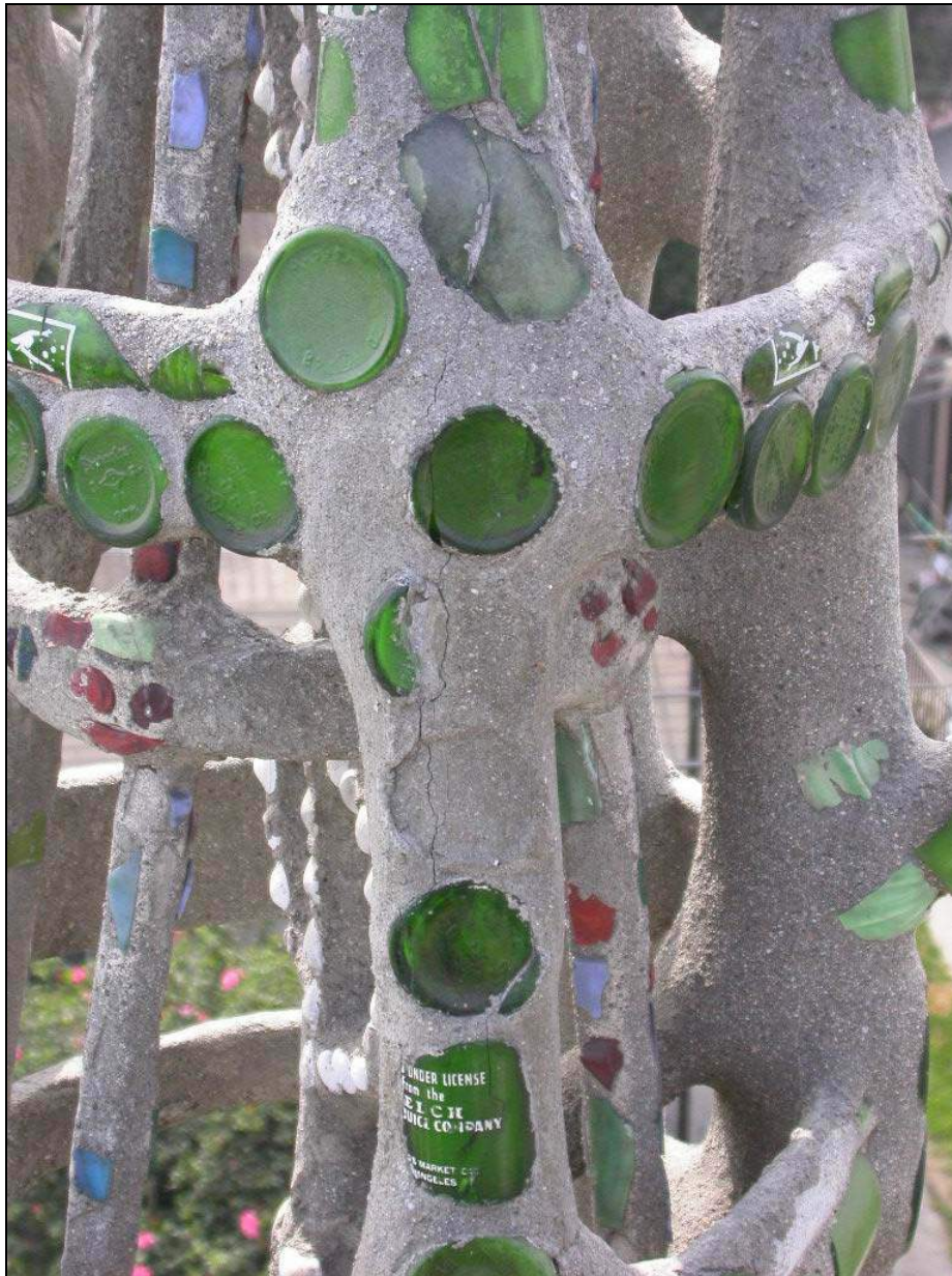
Figure 12: Cracks on East Tower at exterior column through glass embedment.
