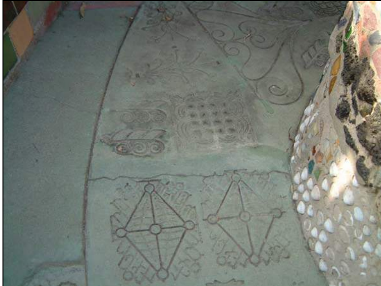
Photo 3. Crack development within sections. The cracks typically occurred perpendicular to the longest axis of the placement.
