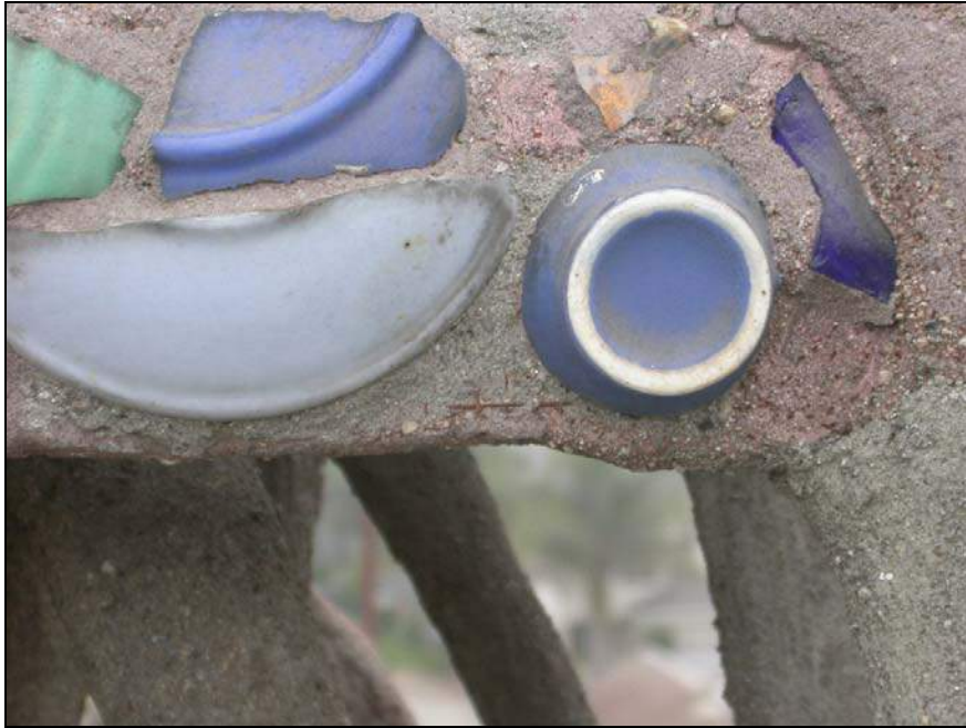
Figure 13: Exposed wire mesh at bottom left of embedded cup on Center Tower.
