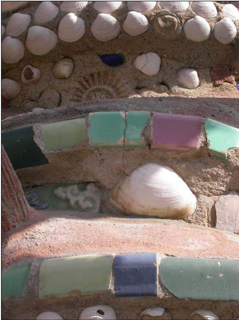
Figure 14: Mock-up no. 5 at center core of East Tower showing crack through mortar and embedded tile before treatment.
