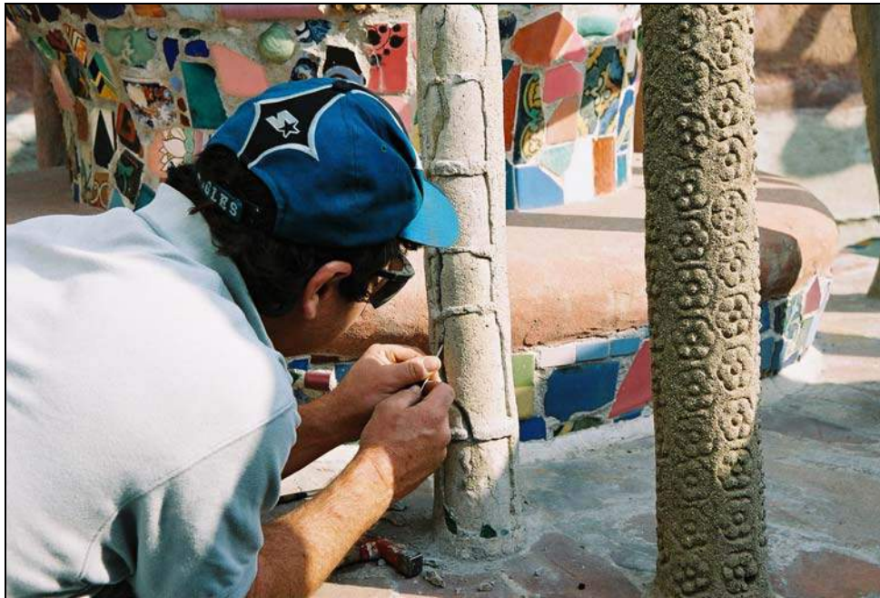
Figure 2: Cutting out of mortar of previous repair using hand tools at mock-up no. 1.
