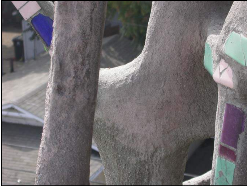
Figure 4: Hairline crack on Center Tower at intersection between exterior column and brace in an area of previous repair.
