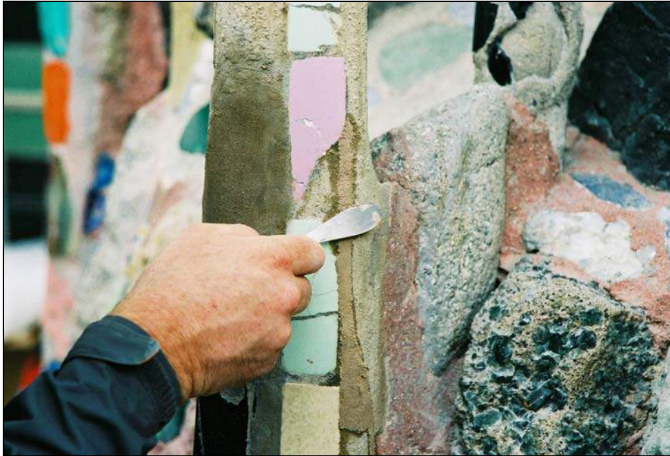
Figure 8: Installation of pigmented Jahn M90 repair mortar at mock-up no. 2.
