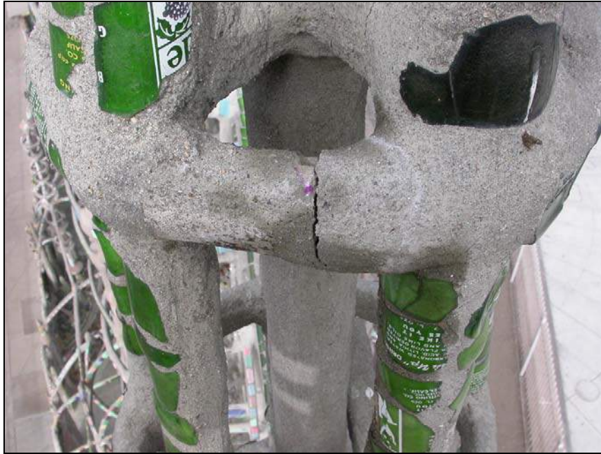
Figure 17: Carbonation test on band of East Tower.
