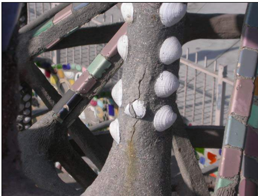
Figure 11: Crack through shell embedding on West Tower at exterior column showing iron staining at bottom of crack.
