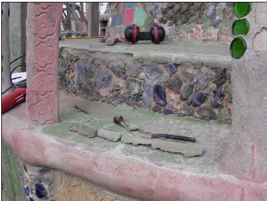
Figure 19: Removed sections of concrete at edge of base level on south side of West Tower.
