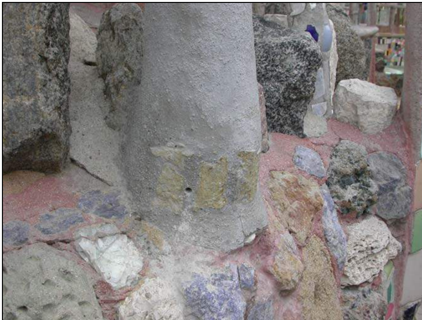
Figure 16: Weep hole at bottom of exterior column at Center Tower.
