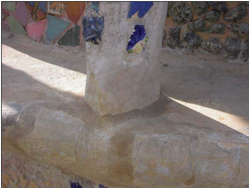
Figure 5: Crazing at previous repair on West Tower at bottom of exterior column.
