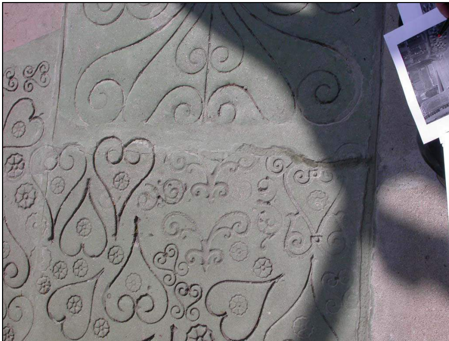
Figure 20: Crack through green colored concrete that has been previously repaired.
