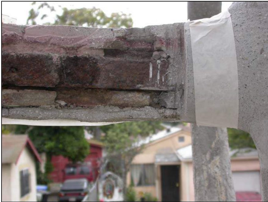
Figure 18: Original steel armature at exterior band on West Tower, as viewed from the interior face.
