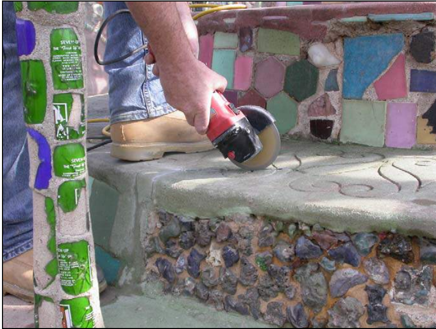
Figure 10: Cutting out of crack at mock-up no. 3.
