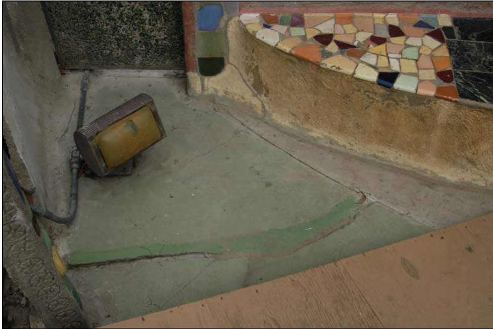
Figure 19: Floor at northwest corner of site showing crack with displacement and previous repair.
