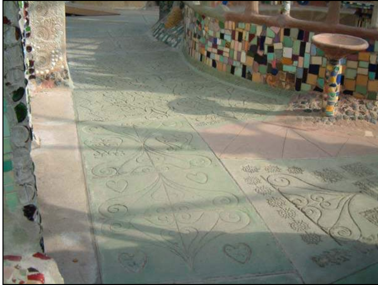
Photo 1. South side of slab near gazebo. The stamp patterns, joint locations and coloring of sections are typical of the entire slab area.
