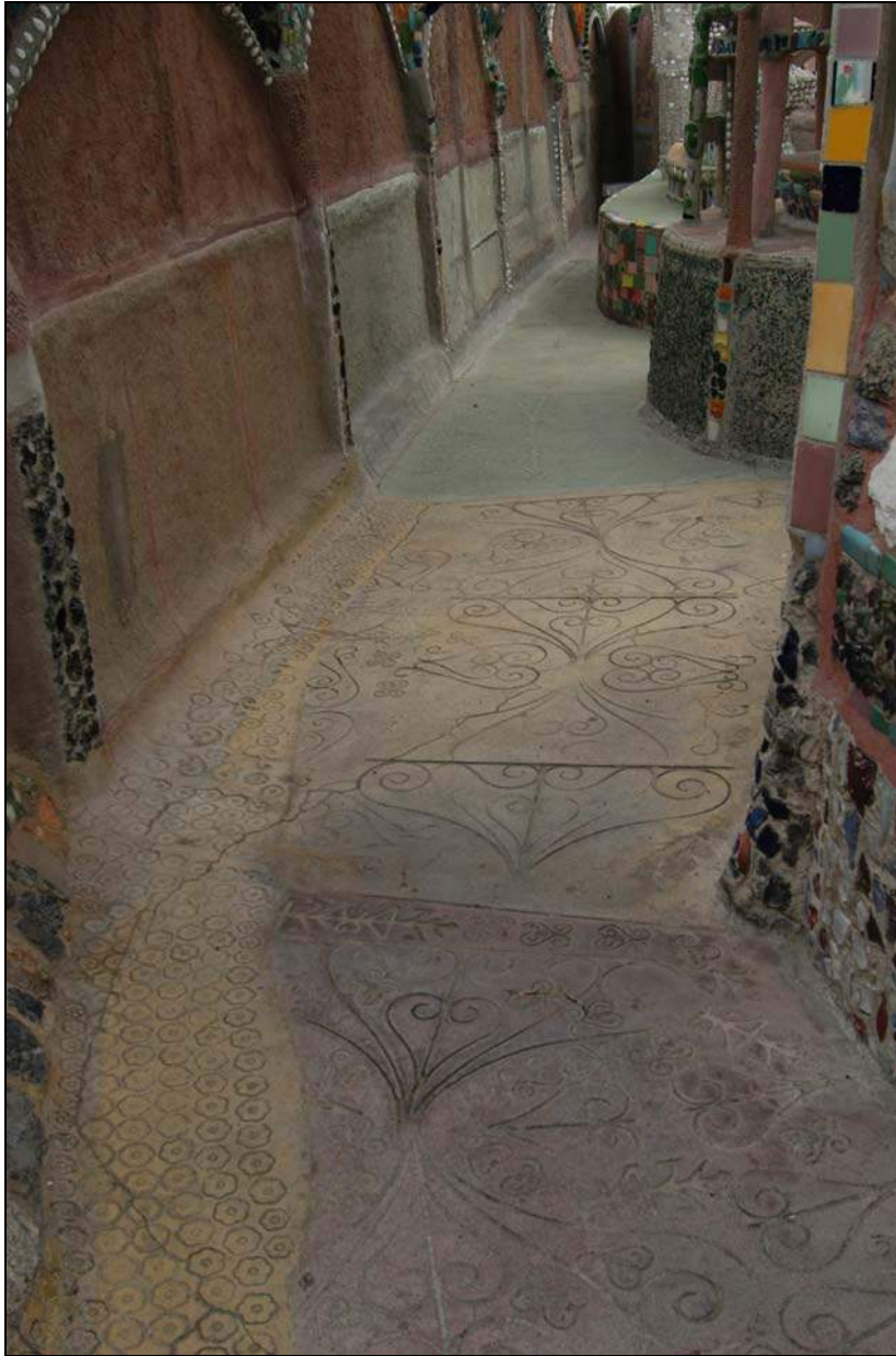
Figure 18: Ornamental floor on the north side of the towers showing red-, yellow-, and green-colored concrete slab with stamped patterns.
