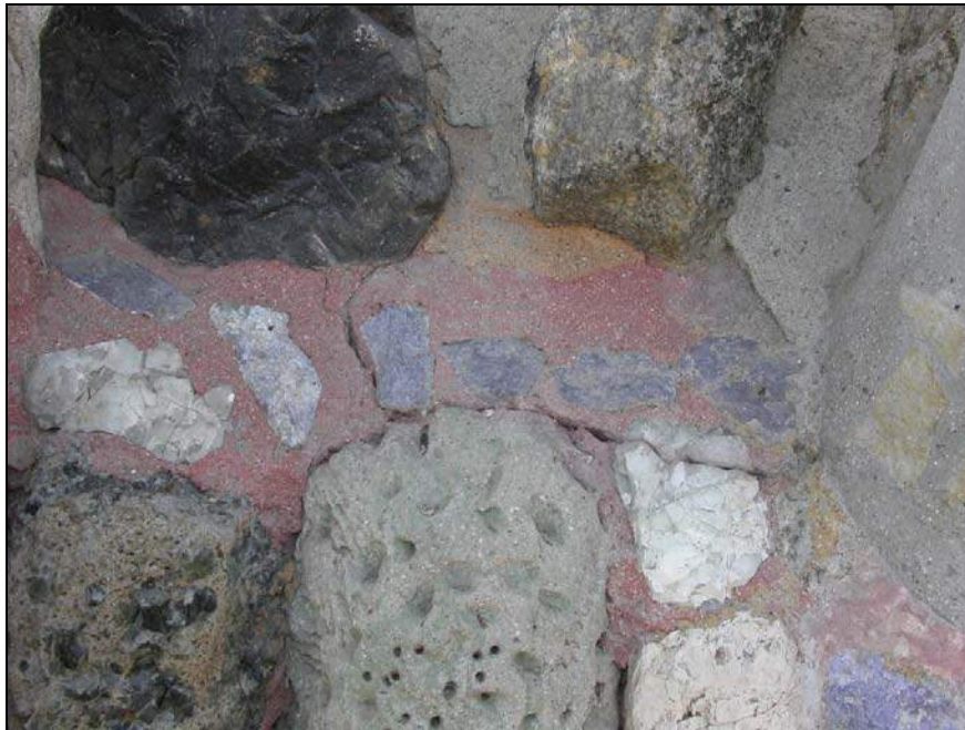
Figure 6: Crack on Center Tower at base.
