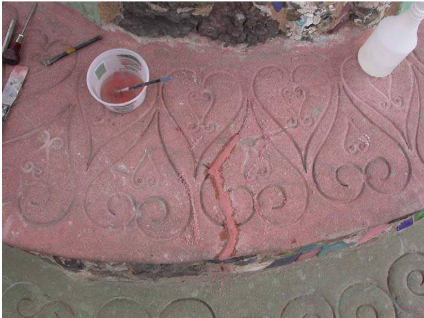
Figure 13: Mock-up no. 4 during installation of pigmented Jahn M90 repair mortar.
