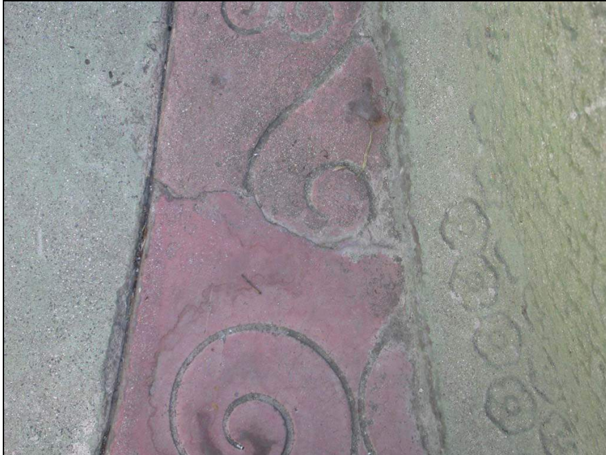
Figure 22: Spall at edge of score line in concrete floor.
