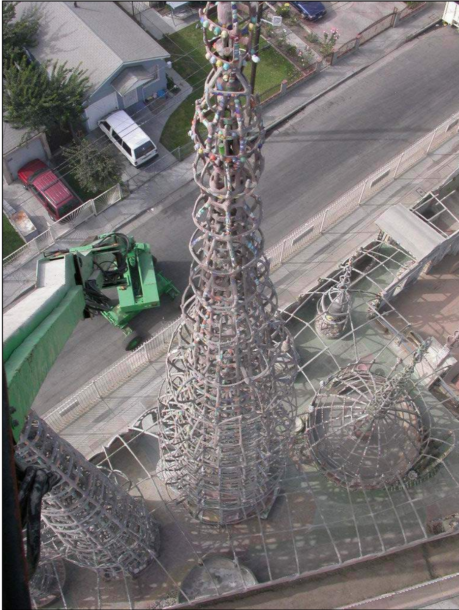
Figure 1: View looking southwest of West Tower from boom lift.
