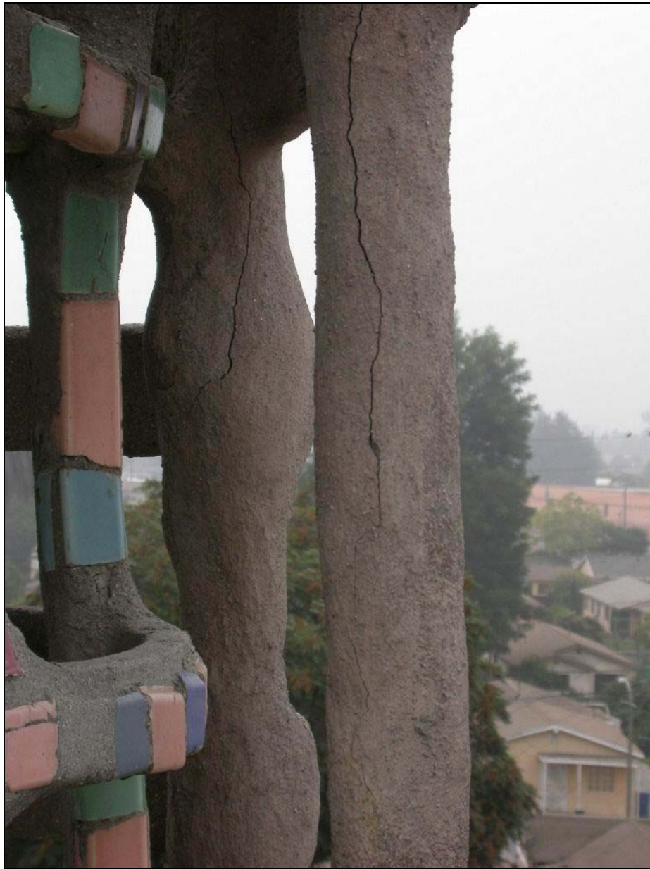
Figure 8: Crack on Center Tower at exterior column in an area of previous repair.
