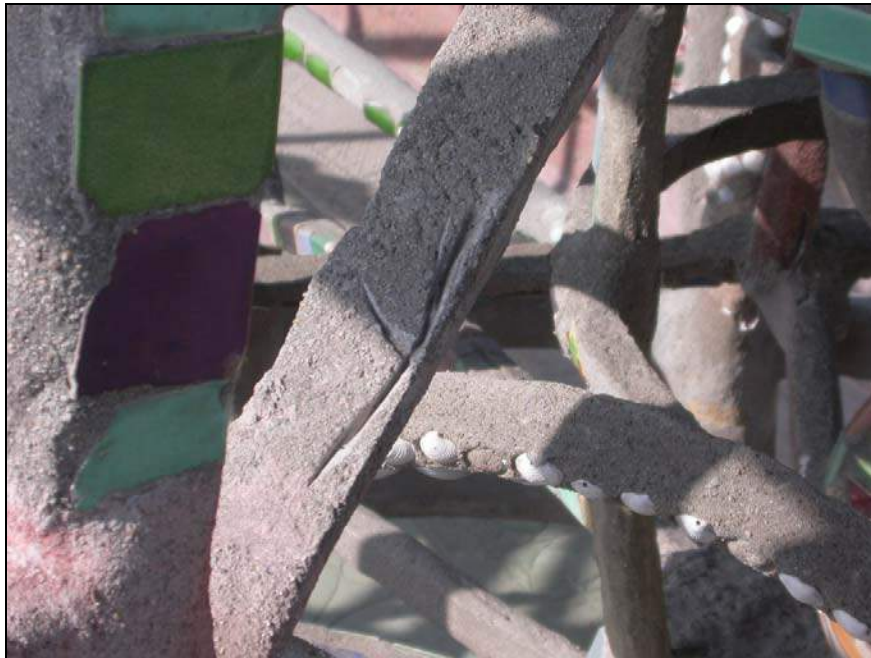
Figure 10: Crack on West Tower at loop that has been partially cut out.
