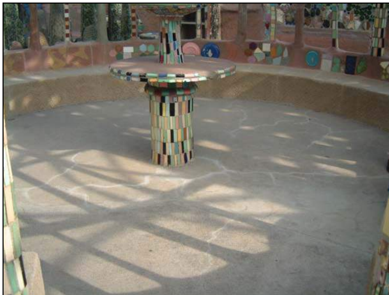
Photo 4. Crack pattern in Gazebo. The area in the foreground of photo had the least amount of cracks and had solid sounding indications. The area in the background (behind pedestal) had a large number of cracks and had hollow sounding indications.
