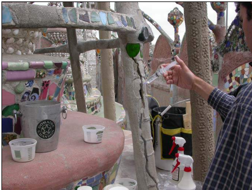
Figure 3: Application of Ferrogard 903 rust inhibitor to cut out crack at mock-up no. 1.
