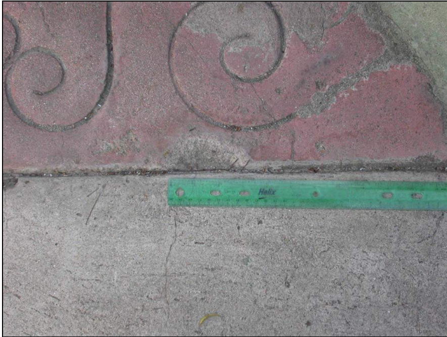
Figure 22: Spall at edge of score line in concrete floor.
