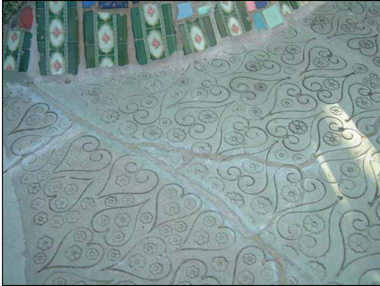
Photo 9. Repaired cracks in west portion of slab just west of West Tower.
