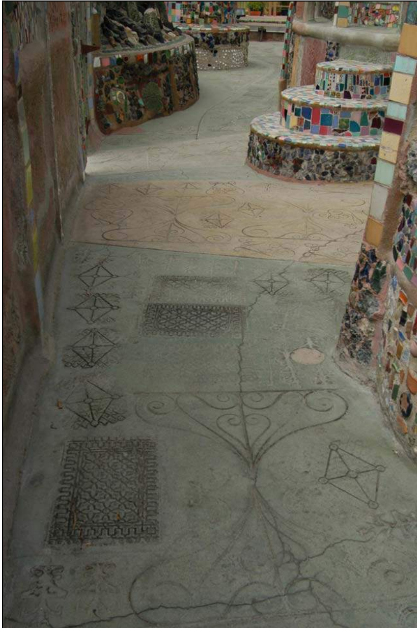
Figure 21: Floor at south side of Center Tower with crack circling the perimeter of the tower approximately 2 feet from the base.
