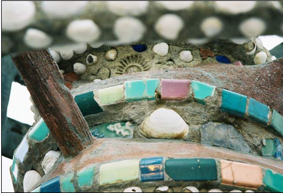
Figure 16: Mock-up no. 5 after installation of Jahn M90 repair mortar at mortar and Edison Coatings Thin-Fill 55 at tile.
