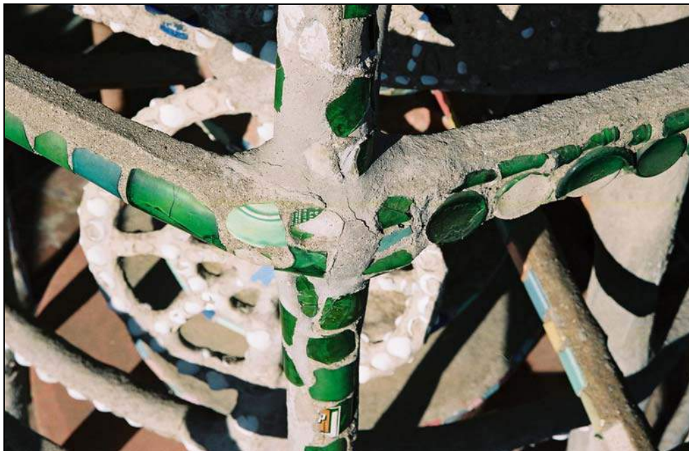
Figure 7: Crack on East Tower at intersection between of exterior column and exterior band.
