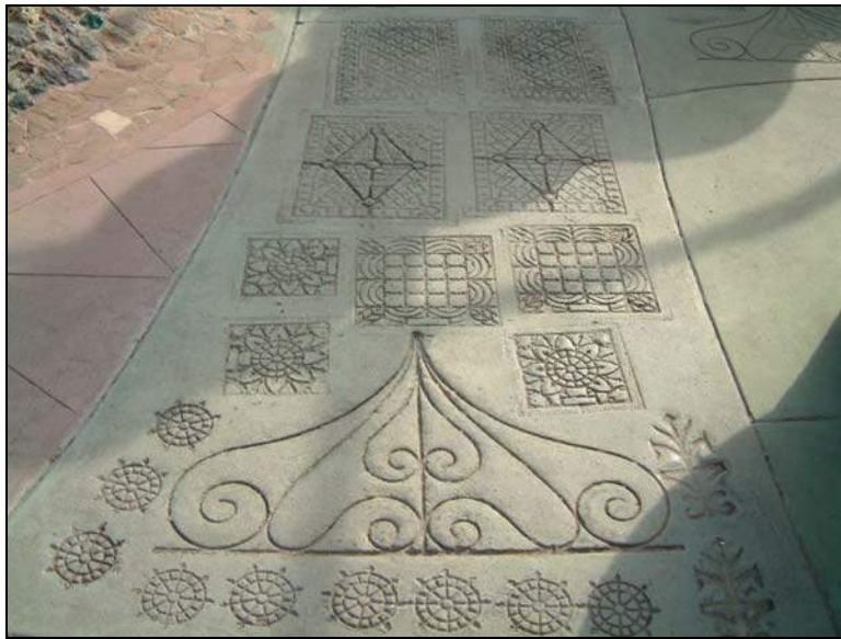
Photo 2. Stamped patterns in walkway.
