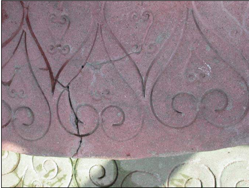
Figure 12: Mock-up no. 4 at west side of red base level of West Tower before treatment.
