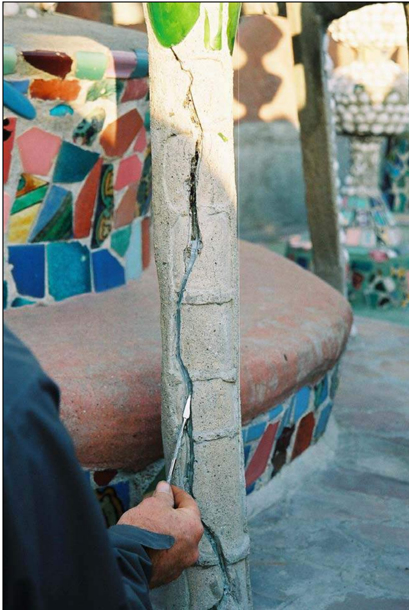
Figure 4: Mock-up no. 1 during application of sealant at middle of crack and epoxy resin at bottom of crack.
