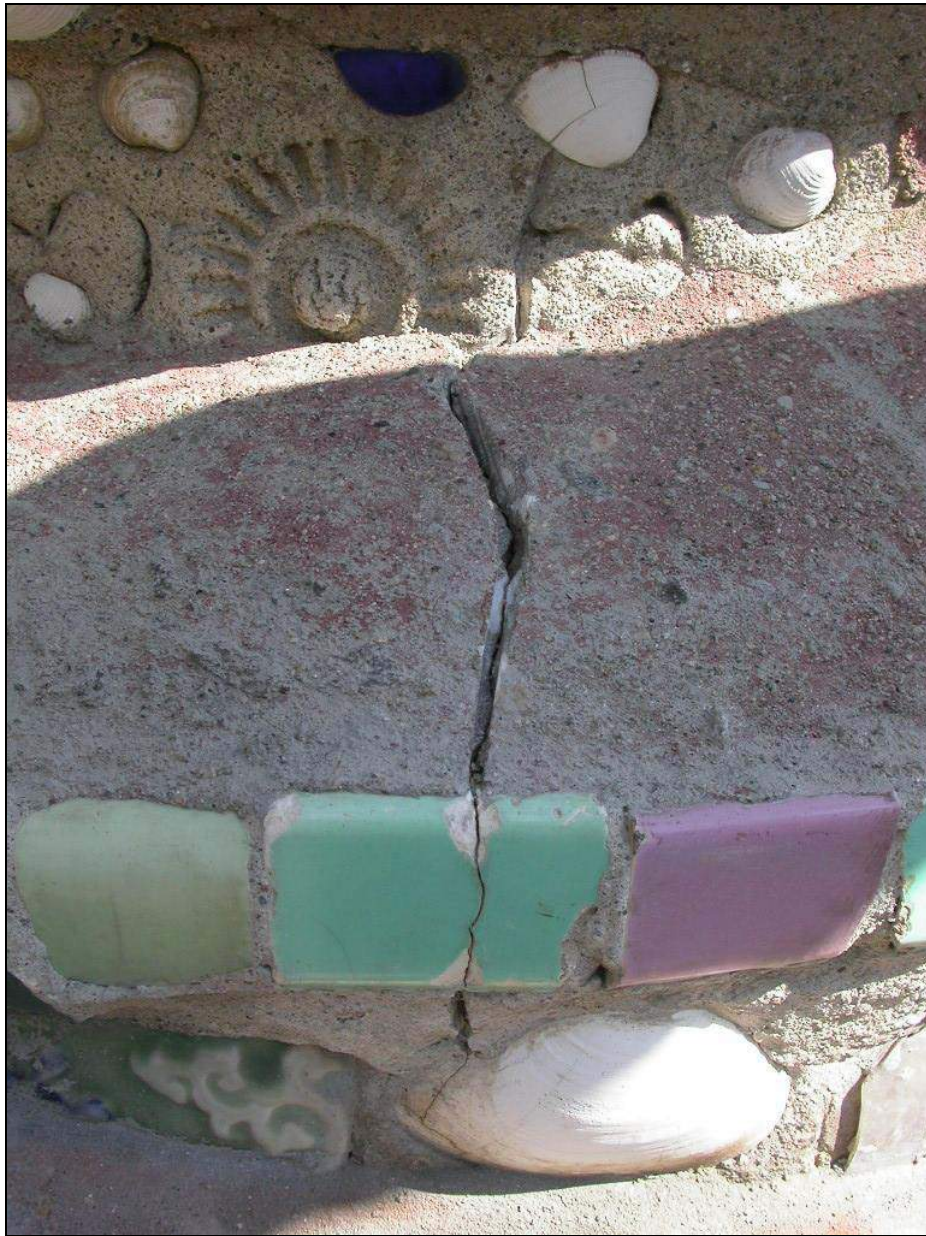
Figure 15: Mock-up no. 5 after cutting out of crack at mortar.
