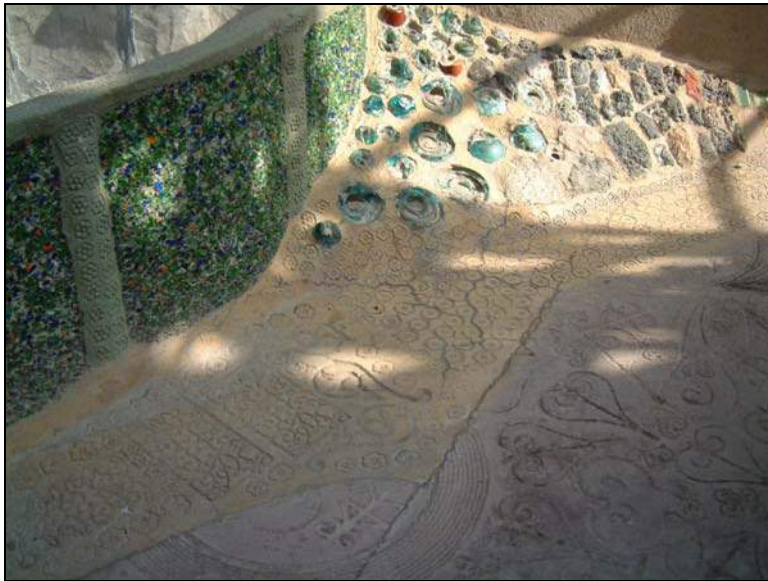
Photo 6. Cracking between color sections in southern portion of slab.
