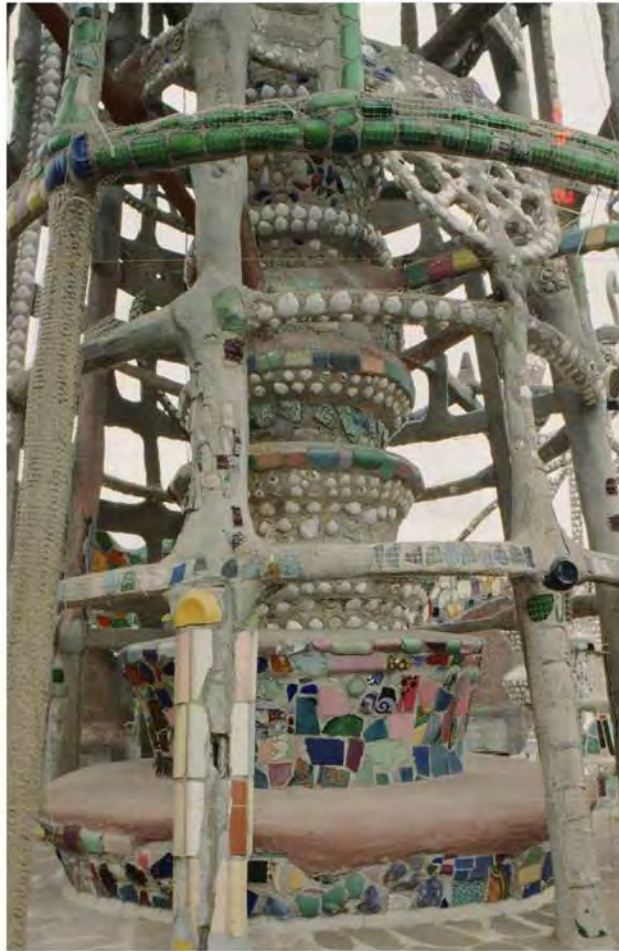
East Tower Columns 4 and 5 1987
