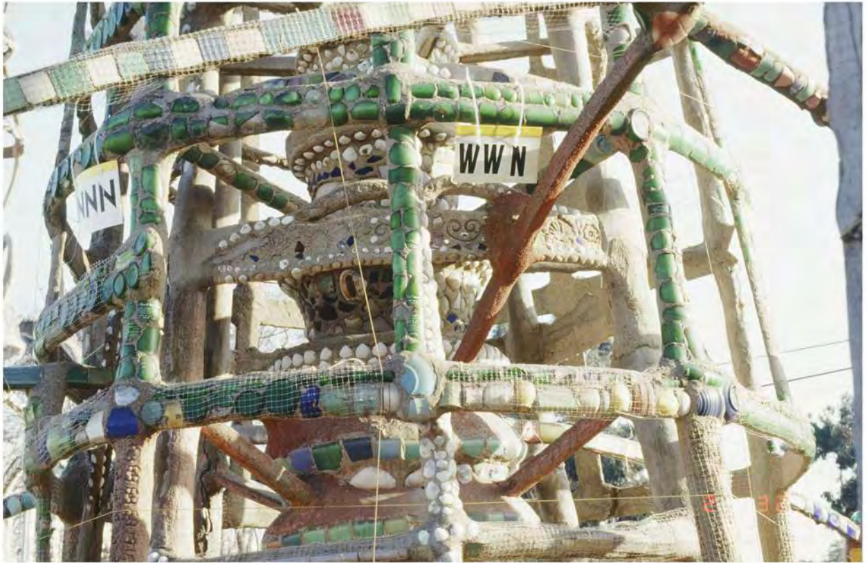
East Tower Columns 5 and 6 1987
