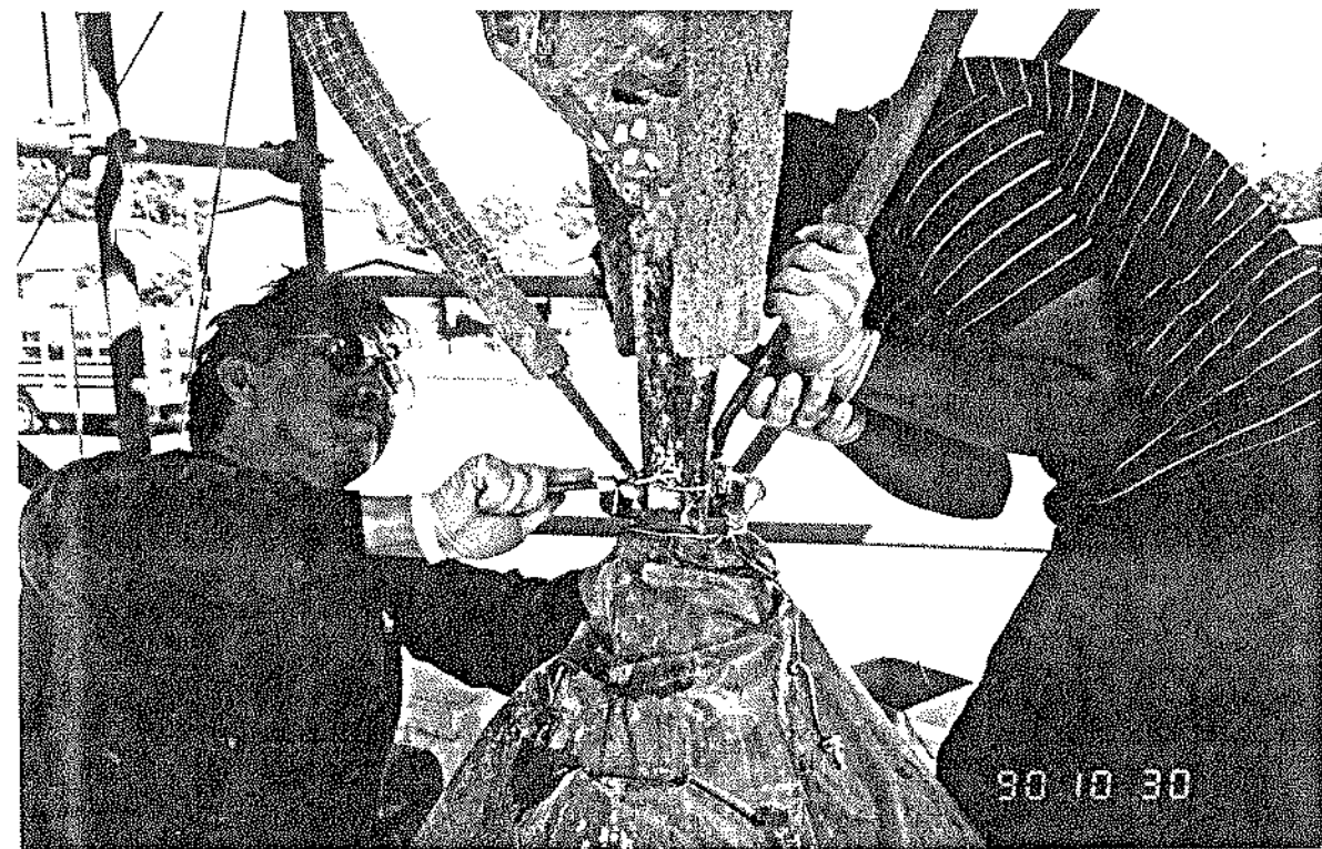
Figure 26. Main spire arc junction under repair and reattachment to central column. Oct 1990.
