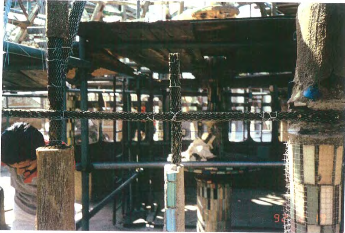
Figure 33. Steel reinforcements wrapped with steel mesh ready to accept mortar and rebonding operation for original covering of mortar and ornaments. Feb 1992.
