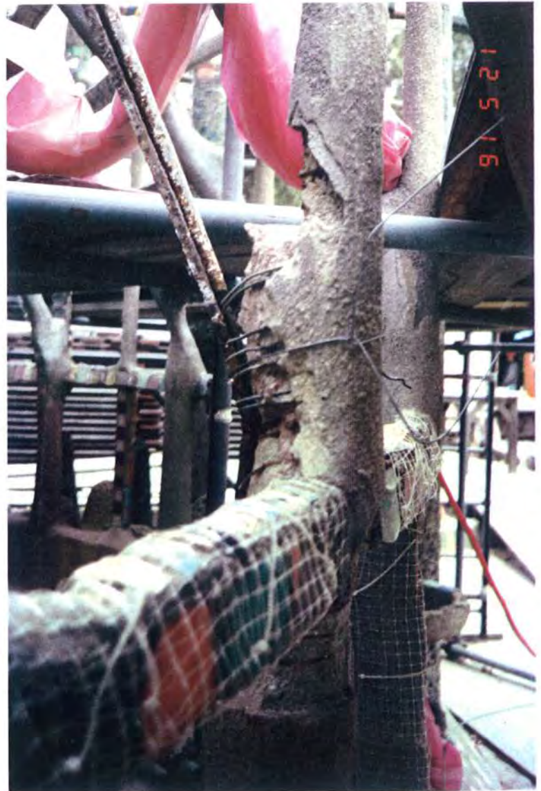
Figure 19. Support MajV02 lower joint with wire attachments exhibiting rust and cracks. May 1991.
