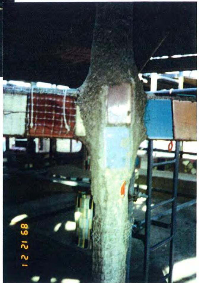
Figure 17. Minor vertical west of Gazebo entrance after crack-filling. December 1989.
