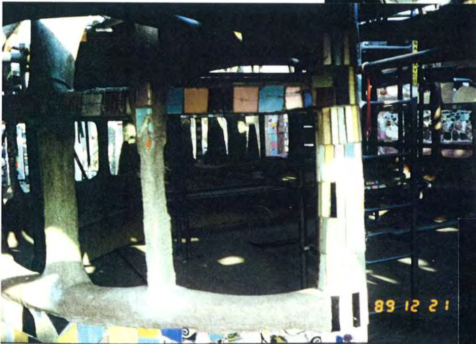
Figure 16. Area west of Gazebo entrance after crack-filling and bonding ornaments to members. December 1989.
