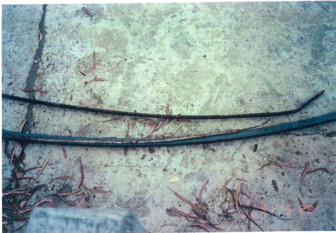
Figure 20. Top-rusted channel, center-rusted rebar, bottom-new 'T' section for MajV02 reinforcement before installation. May 1991.
