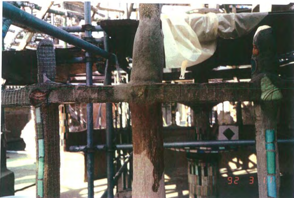
Figure 34. Application of final coat of mortar and rebonding of original covering of mortar and ornaments. Mar 1992.
