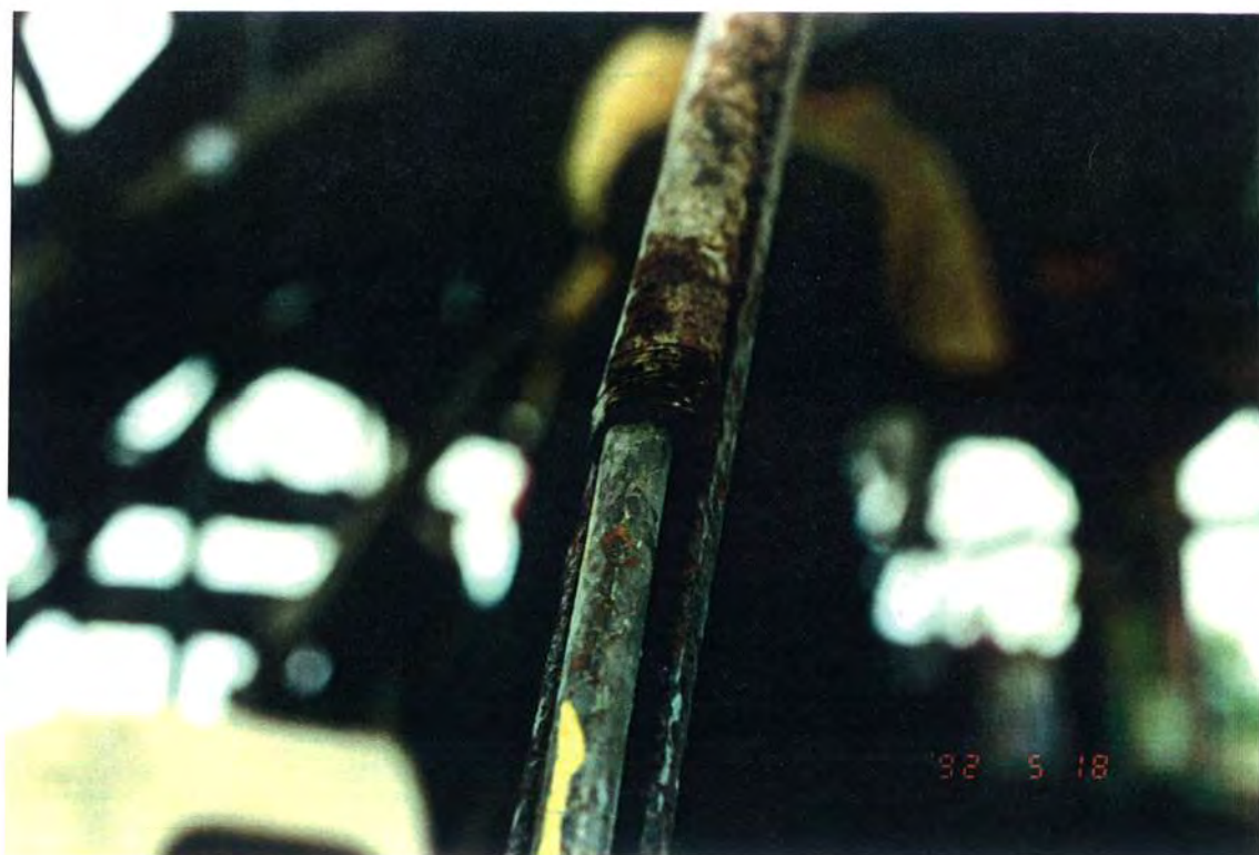
Figure 14. Major vertical support rein- forcement by Rodia. Pipe nested in channel on top with rebar inserted in pipe on bottom of photo. May 1992.
