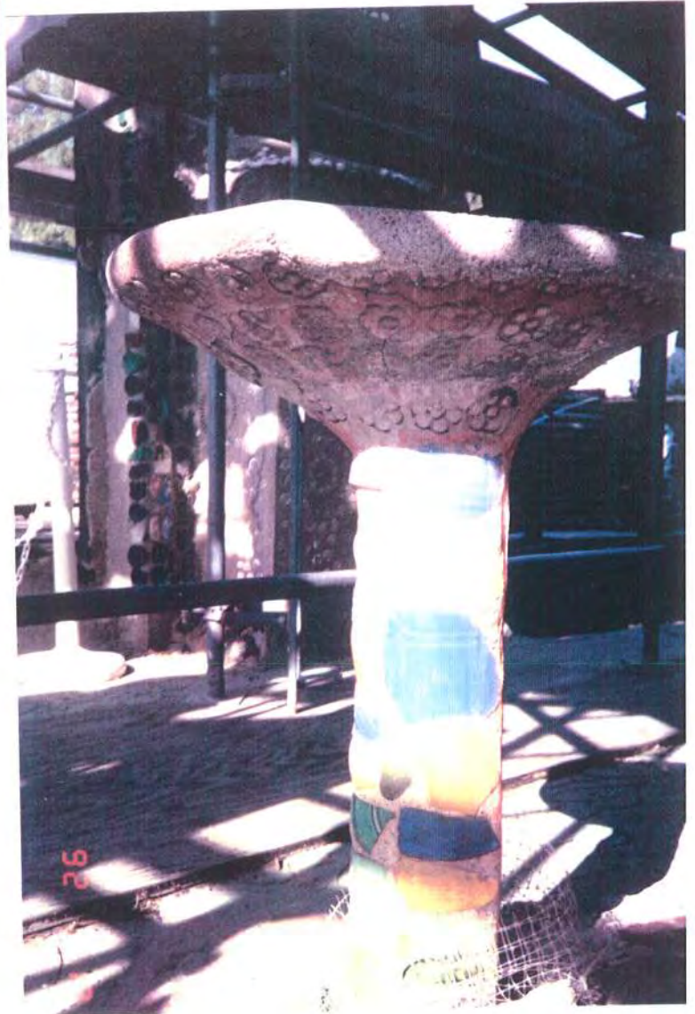
Figure 30. Damaged birdbath southwest of Gazebo. Jan 1992.
