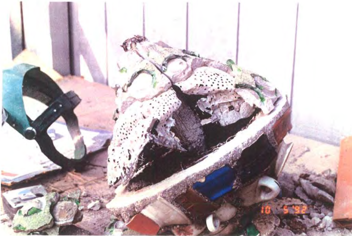
Figure 28. Finial opened, showing one of two colanders used to form the upper and lower portions of the finial. Oct 1992.
