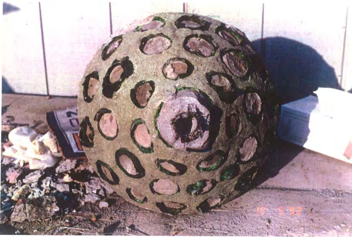
Figure 27. Finial from top of damaged outer vertical after removal. Oct 1992.
