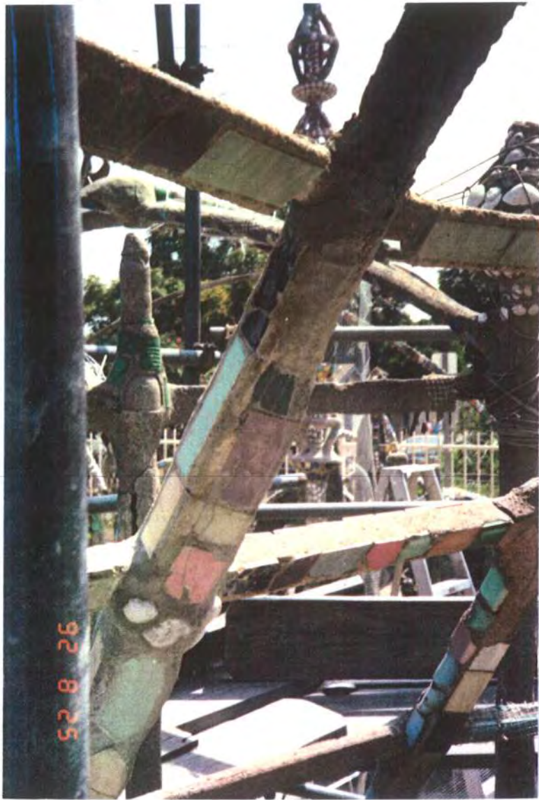
Figure 37. Third arched support after rebonding of original covering. Aug 1992.
