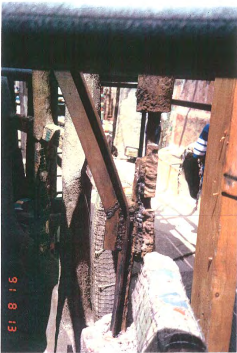
Figure 29. Lower attachment of first 'T' section support after welding to horizontal band and outer vertical steel reinforcements. Aug 1991.
