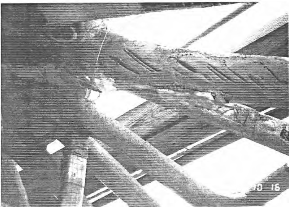
Figure 24. Top of photograph shows support MajV02 after repair mortar application over new 'T' reinforcement. Oct 1991.
