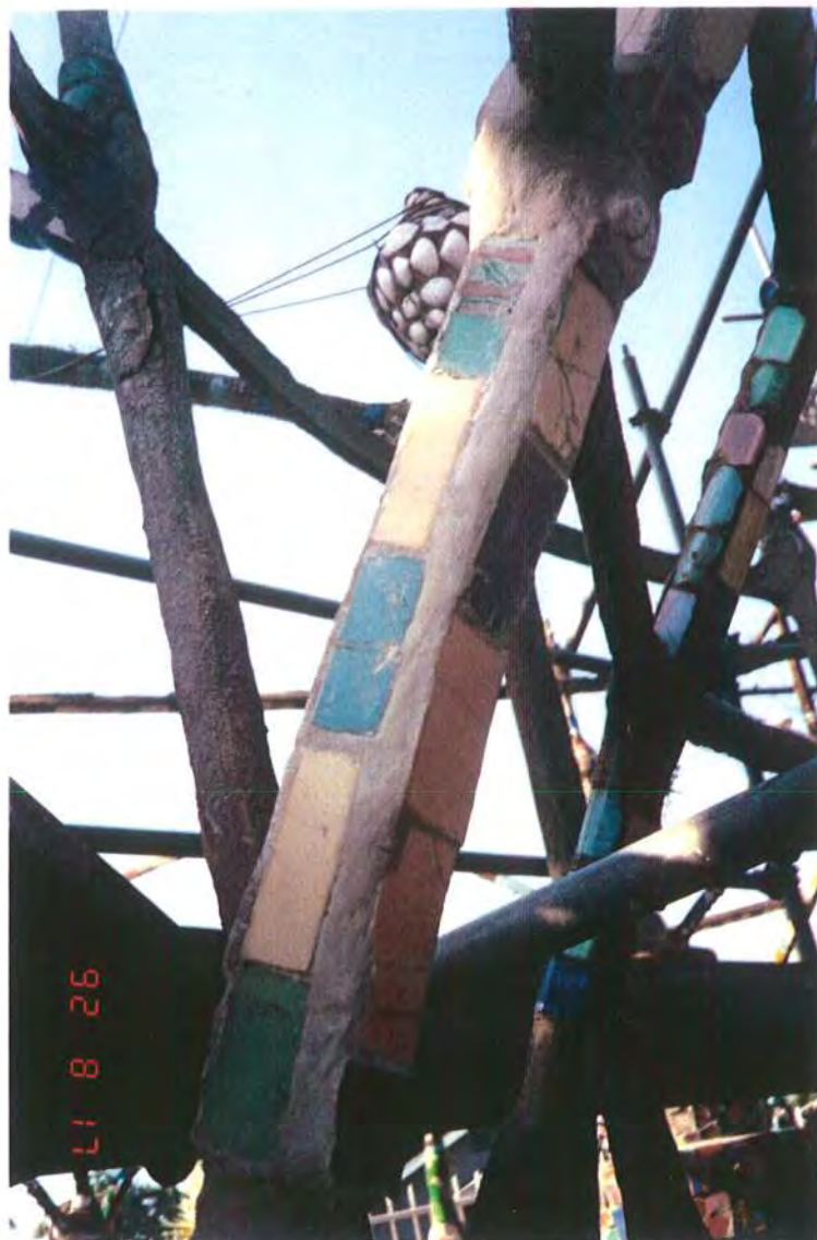
Figure 36. Third arched support after rebonding of original covering over new steel 'T' section reinforcement. Aug 1992.
