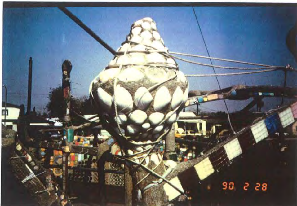
Figure 26. Finial on top of outer S.E. vertical after shell treatment and stabilization. Feb 1990.
