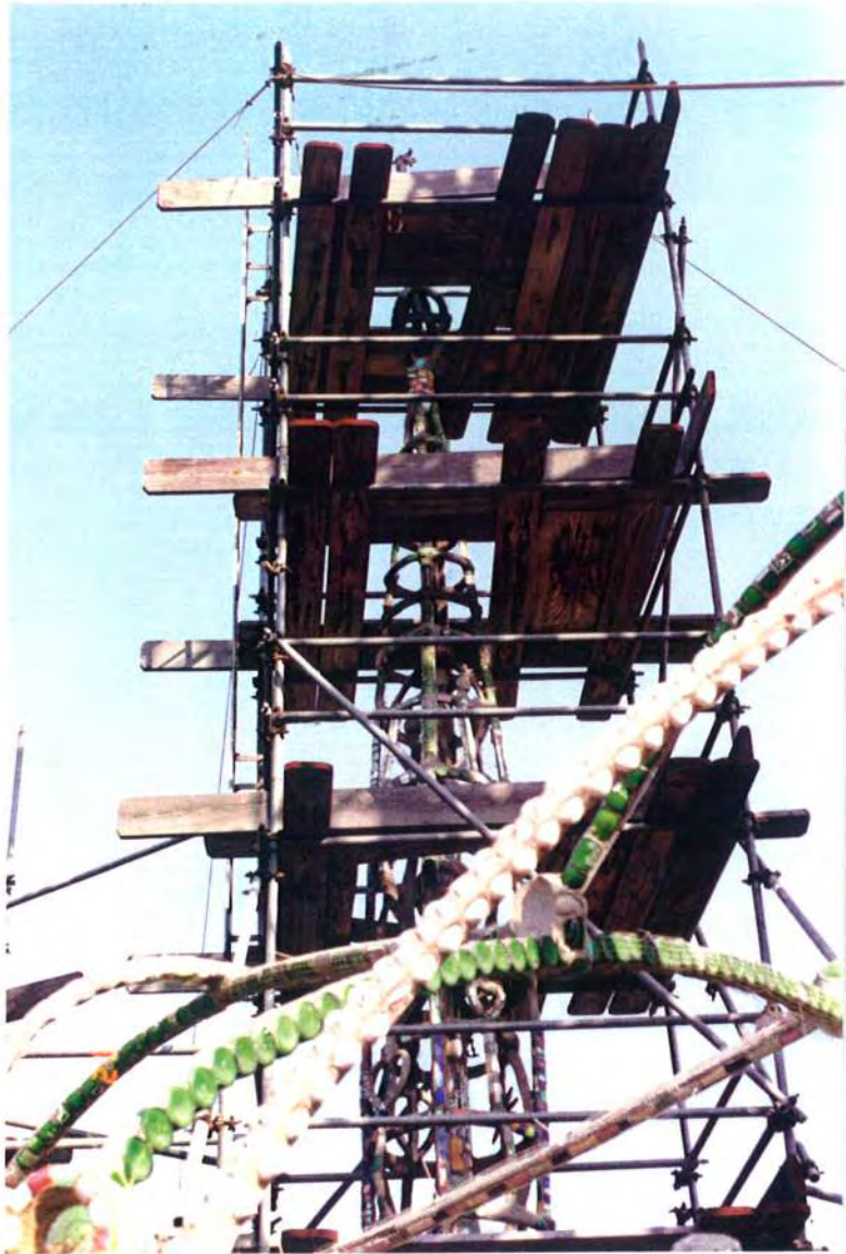
Figure 9. Scaffolding around Gazebo spire for conservation program access. Oct 1992.
