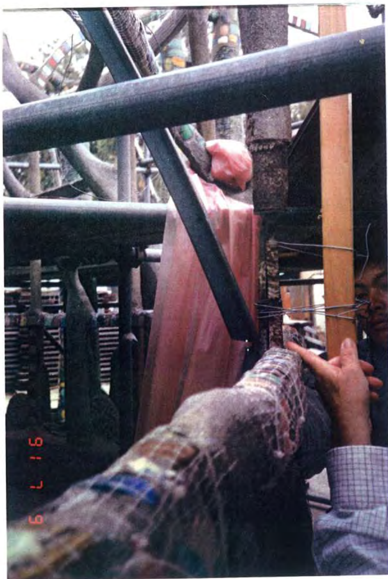
Figure 21. New 'T' section in place for welding at lower end to verti- cal and horizontal band. Jul 1991.
