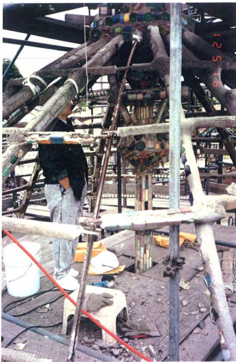
Figure 18. Support MajV02 after removal of cover showing rusted channel and rebar nested in channel. May 1991.
