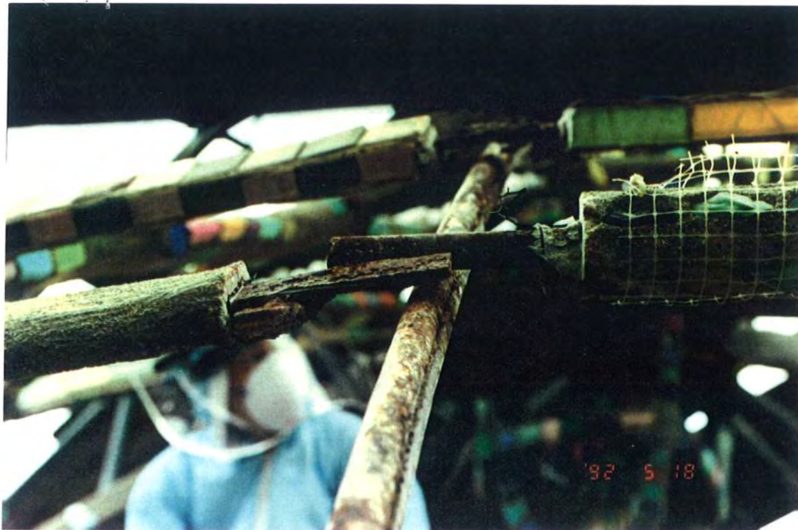
Figure 13. Junction of horizontal bands with major vertical support. May 1992.
