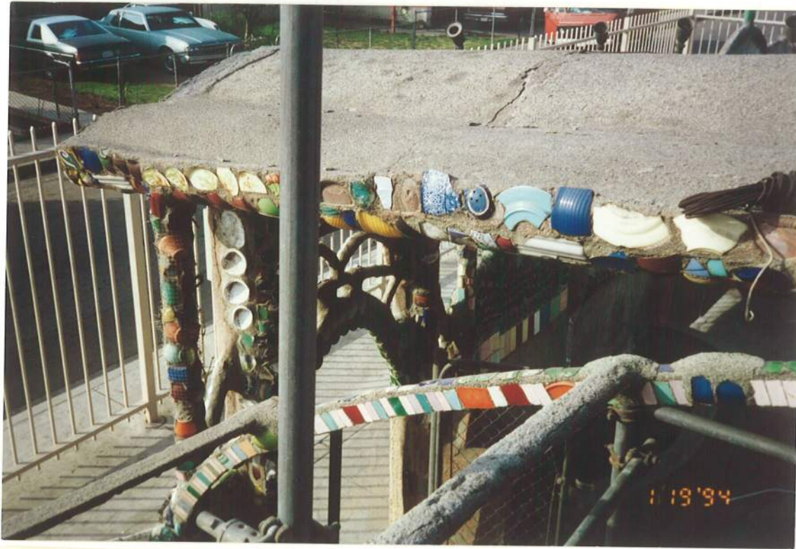
Figure 4. Canopy sculpture top showing cracking failures after January 17 Northridge earthquake. Looking northeast from above. January 19, 1994.
