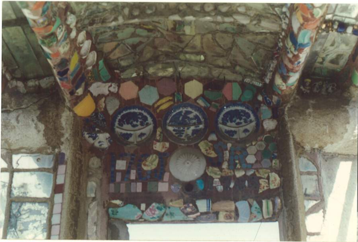
Figure 6. Canopy (top) over ornamentation on House Facade above front door. Looking north from entry. November 1993.
