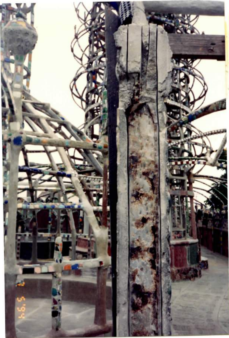
Figure 23. House facade outside (south) west end of facade during crack-filling with Jahn mortar. July 5, 1994.
