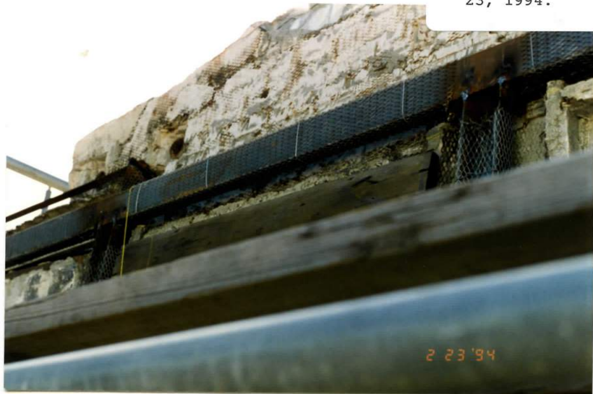
Figure 17. Inside (north) facade horizontal steel channel replacement for damaged top beam. Note top beam welded to new vertical channels on both sides of door opening. February 23, 1994.
