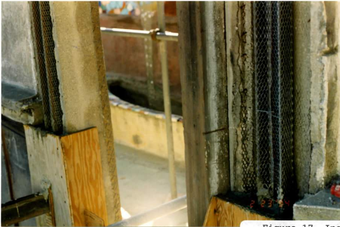
Figure 17. Inside (north) facade horizontal steel channel replacement for damaged top beam. Note top beam welded to new vertical channels on both sides of door opening. February 23, 1994.
