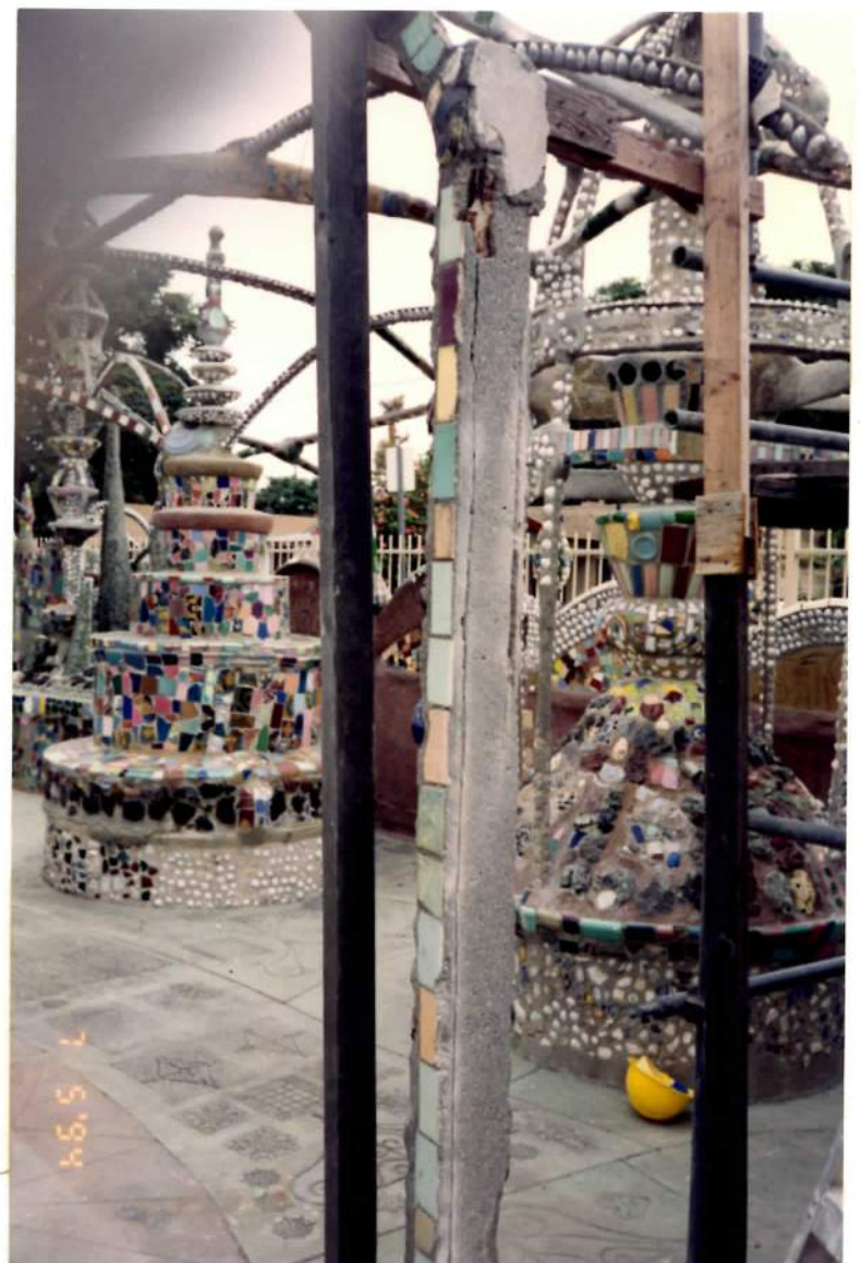
Figure 21. Post 08 east of house foundation showing vertical cracks and damage at top near connection to overhead. July 5, 1994.
