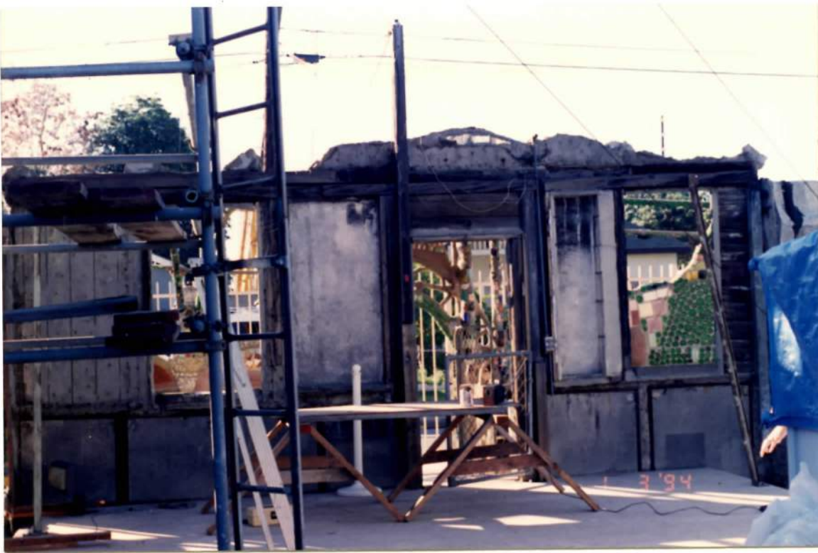
Figure 8. Inside (north) elevation of facade. January 3, 1994.
