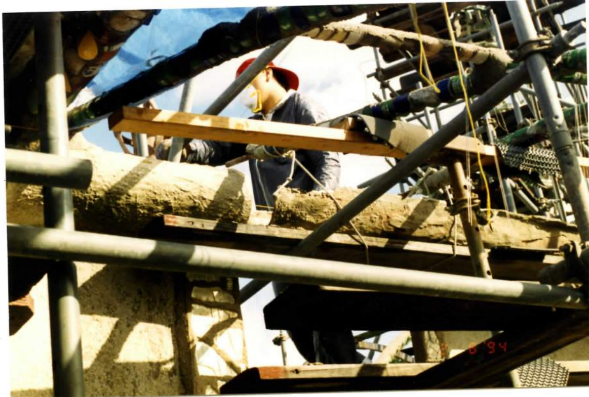
Figure 14. Removal of portion of facade top beam outside (south) before conservation. February 8, 1994.
