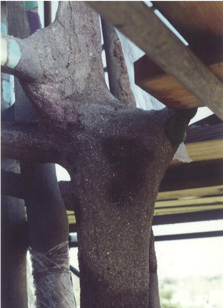
Upper photo shows exposed columns where damaged band #19 has been removed prior to installation of new steel channel. Wood beams support the upper ring to compensate for reduced strength in columns. February 1996.
