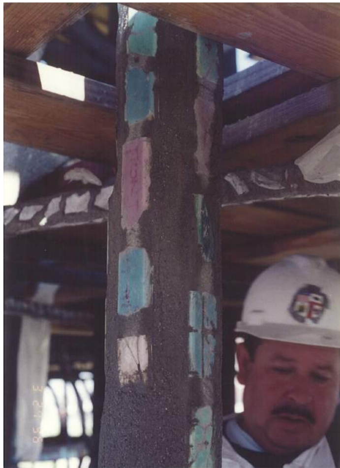
Completed vertical columns. Ornaments had been covered by subsequent applications of repairs by Rodia and/or State. May and August 1996.
