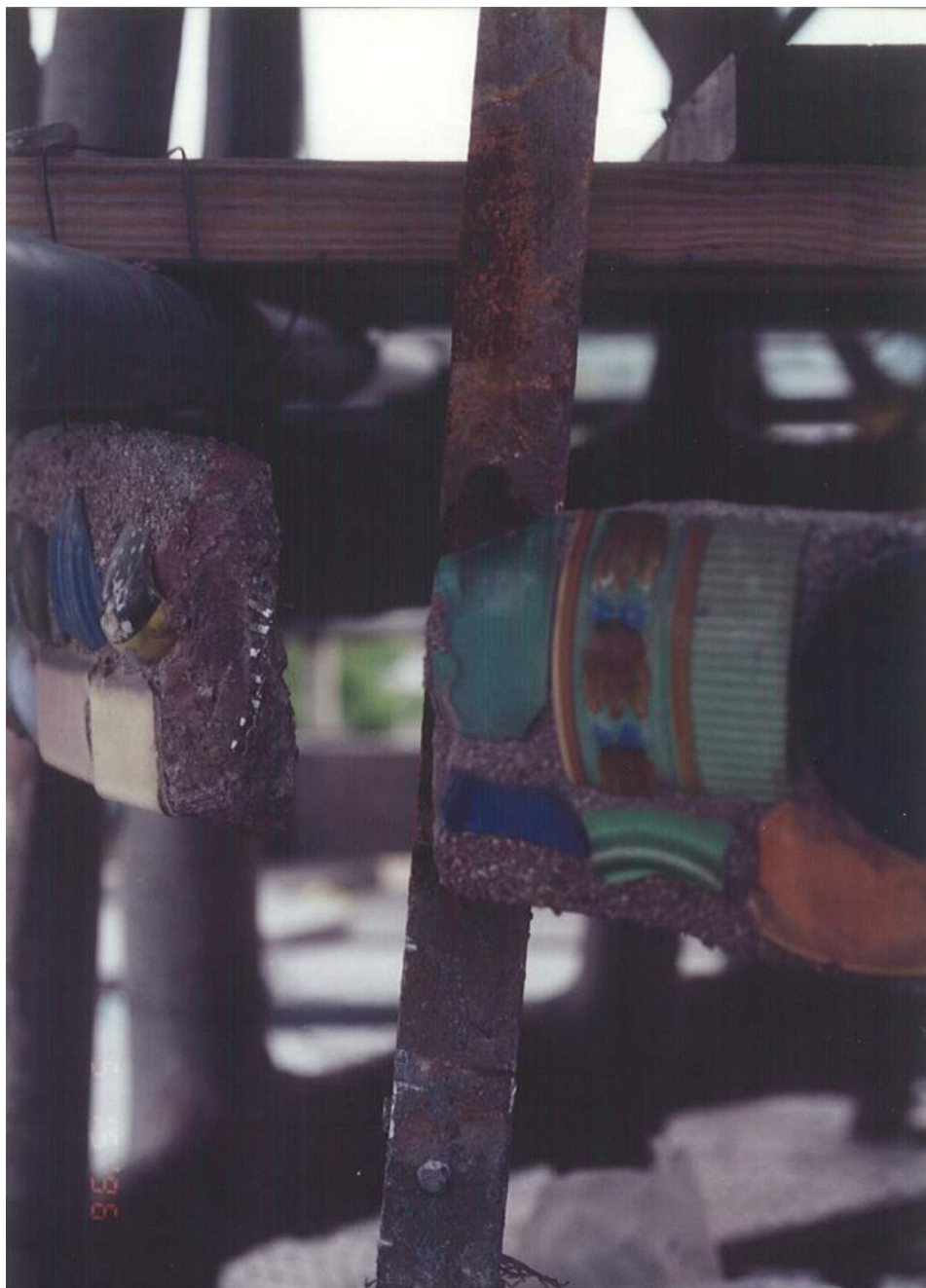
Repairs in progress. Exposed wire ends within horizontal band, left center of photograph and angle reinforcement in vertical column, center of photo. May 1996.
