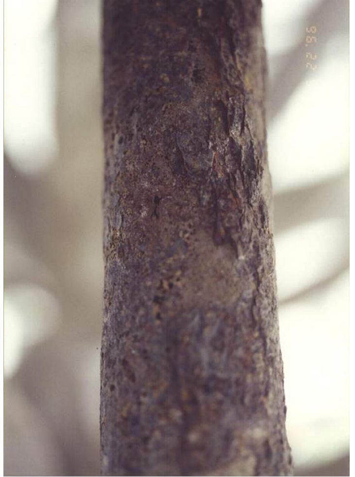
Original column and band reinforcement after opening failed coverings. May 1996
