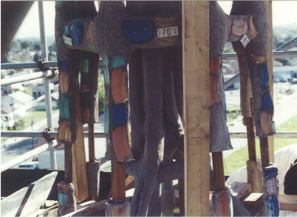
Upper photo shows exposed columns where damaged band #19 has been removed prior to installation of new steel channel. Wood beams support the upper ring to compensate for reduced strength in columns. February 1996.
