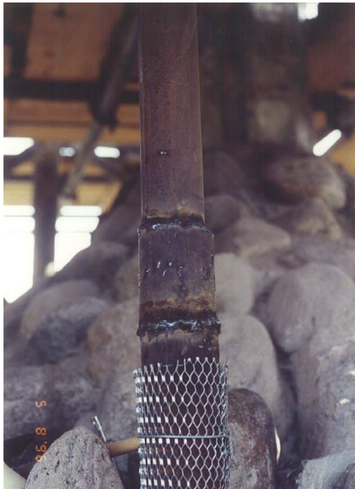
New steel reinforcement installed in Center Tower above base. Mesh has been wrapped around the pipe (left photo) and the pipe has been welded to another pipe directly above it (right photo). May 1996.
