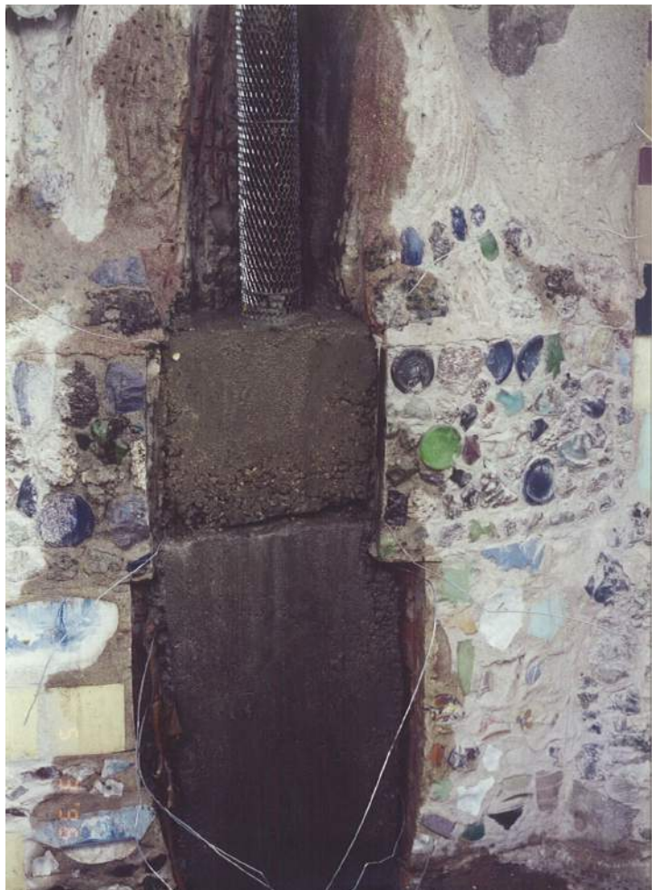
A new reinforcement was installed and welded to the original steel protruding from the base. Mesh was wrapped around the reinforcement and cored with cement mortar. Bottom photo. May 1996
