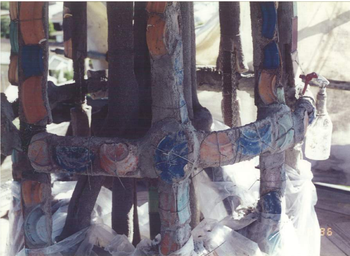
Band repair in progress. Rodia's coverings over each of the band segments are being reinstalled. New mortar was applied over the new reinforcement. Segments had been removed to install the new channel reinforcement. The segments were cut with a diamond cutter. Next they were thinned from the inside to maintain the original overall dimensions and now they are shown reinstalled over new cement mortar coverings. March 1996.
