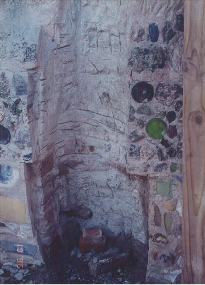
A portion of the Center Tower base was opened to remove a damaged vertical column. Top photo. April 1996.
