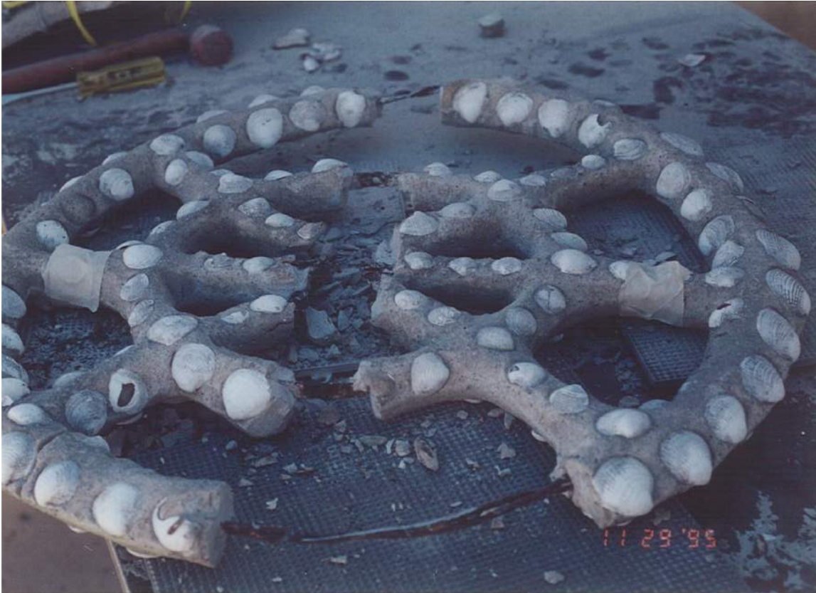
This damaged mortar wheel was removed from the sculpture and repaired on the ground. The upper photograph (Nov. 1995) shows the inside of the wheel under repair. The side of the wheel has fewer damage sea shells than the other side which faces 107th street and suffered vandalism.
