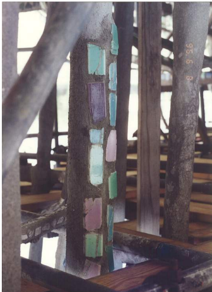
Completed vertical columns. Ornaments had been covered by subsequent applications of repairs by Rodia and/or State. May and August 1996.
