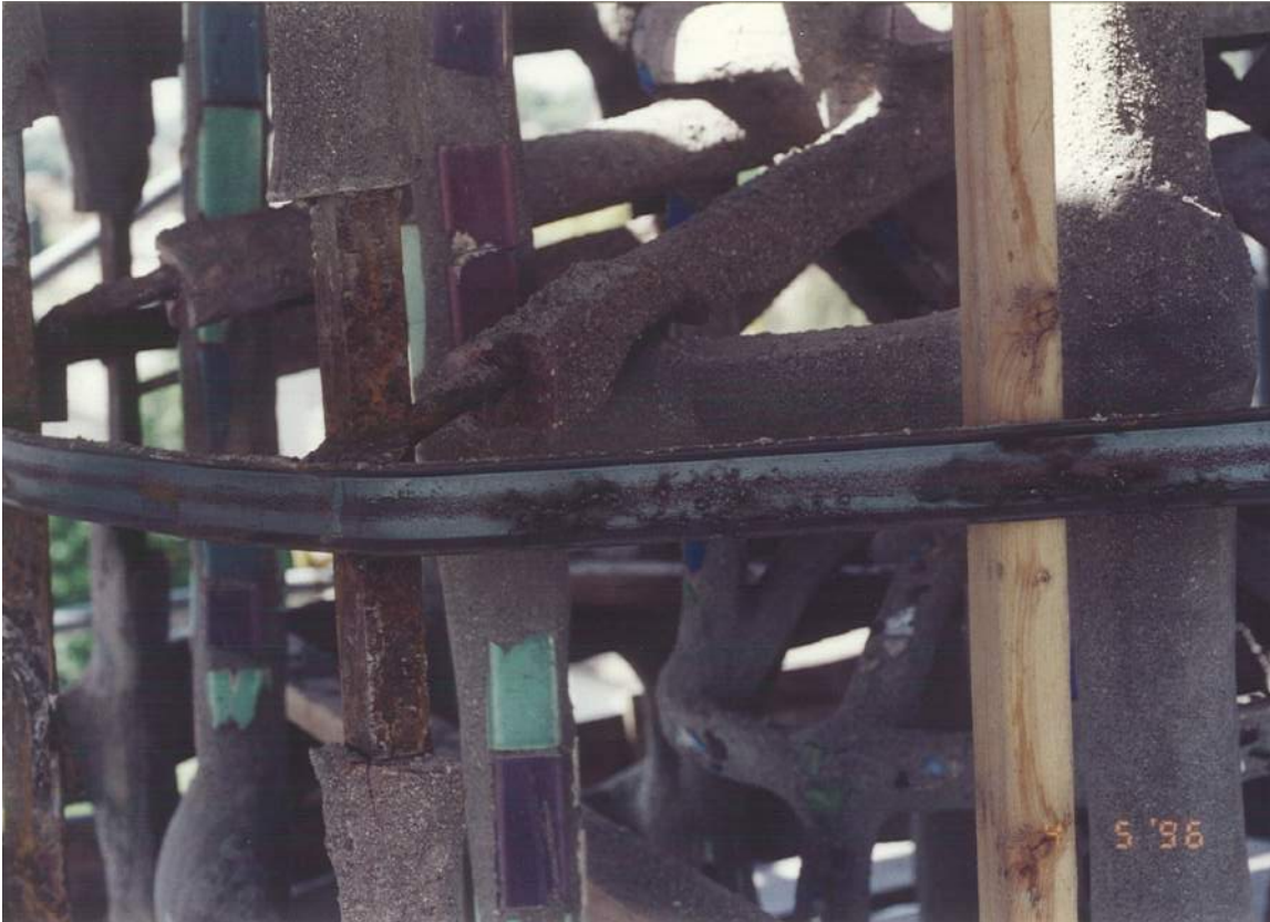
Repair in progress. New channel reinforcement for failed horizontal band and attachments design for columns to the band reinforcement and radials on the Center Tower. April 1996.
