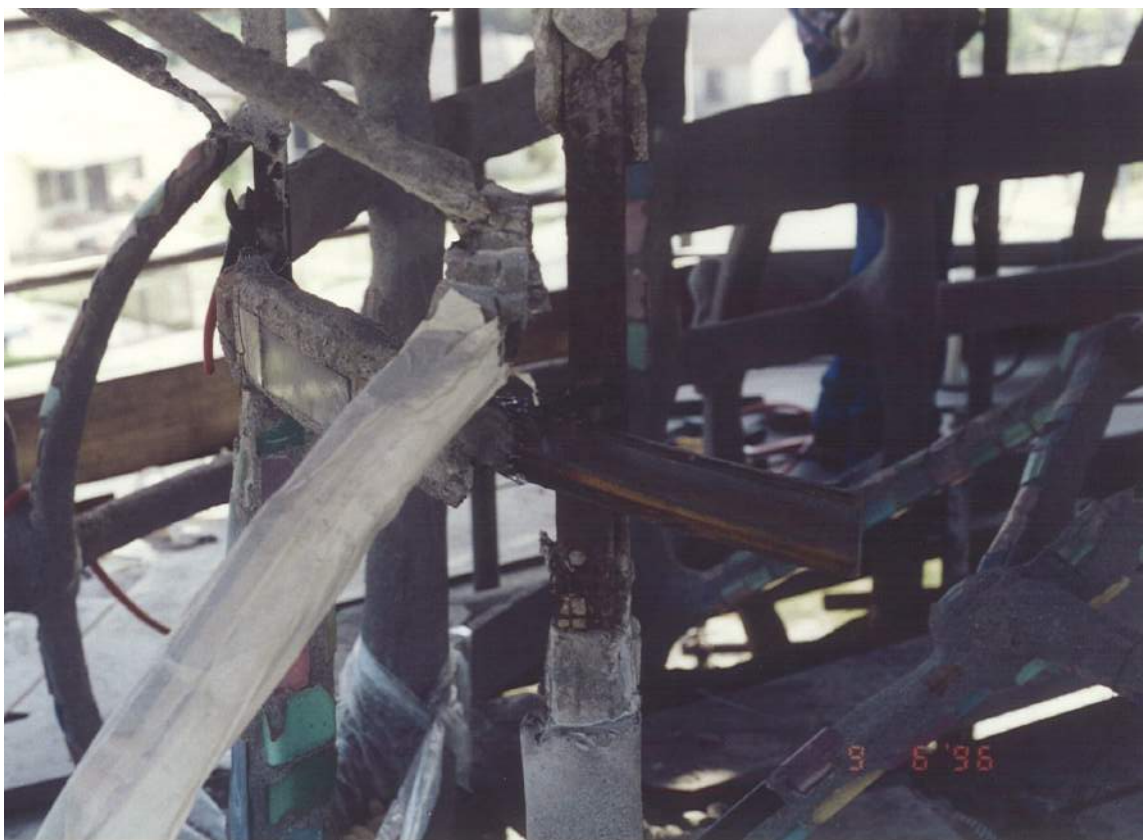
Repairs in progress on horizontal band and joints with vertical columns, radials to the center column and to outer arcs on the West Tower. September 1996.
