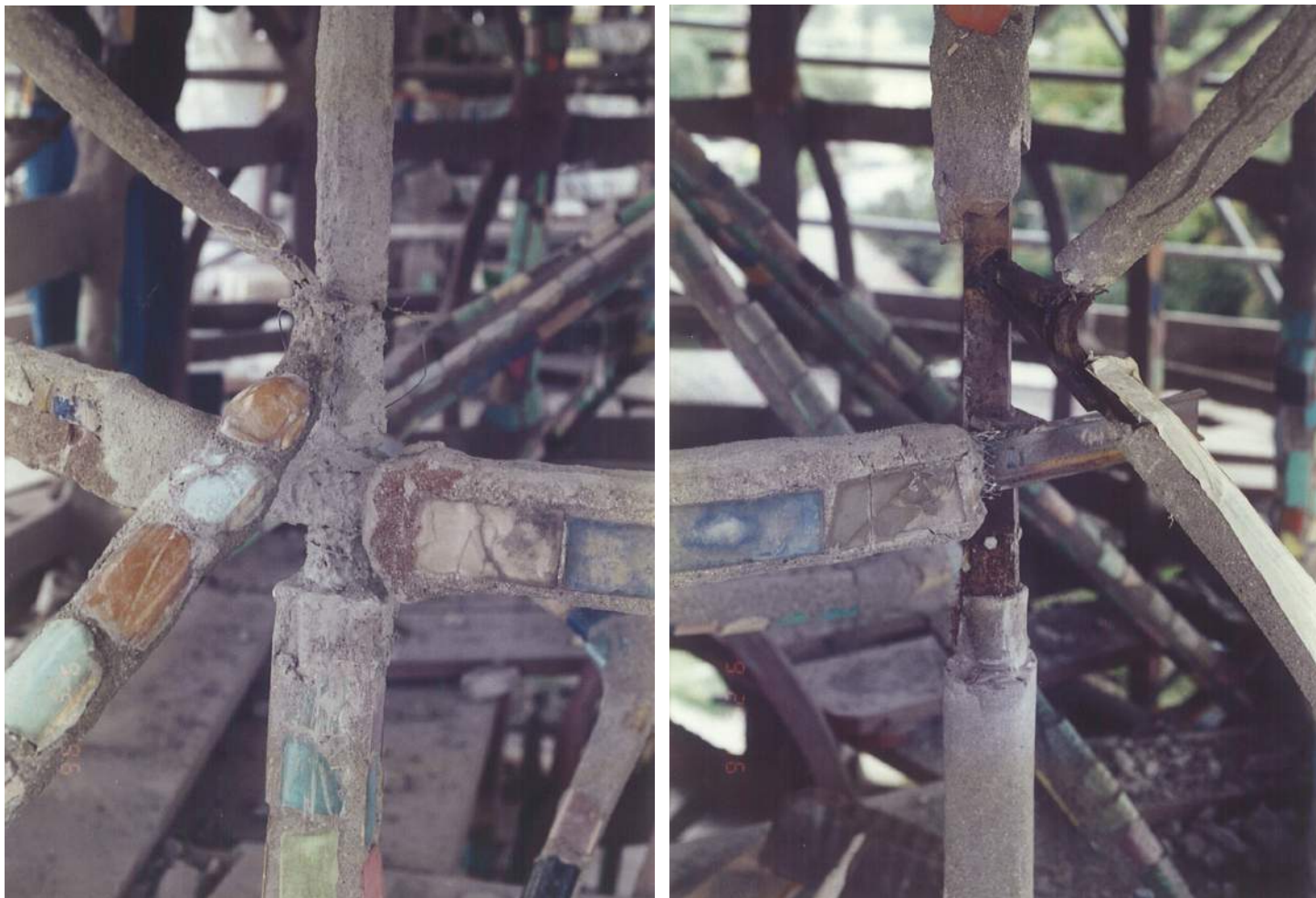
Repairs in progress on horizontal band and joints with vertical columns, radials to the center column and to outer arcs on the West Tower. September 1996.
