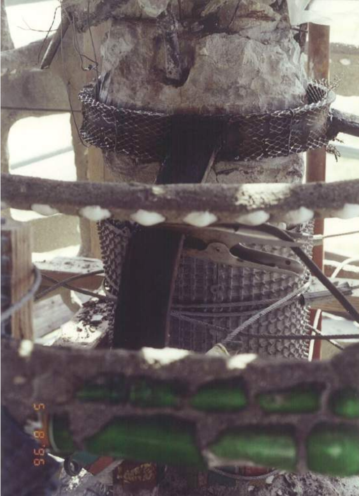
East Tower damage required repairs or replacement of reinforcements in five of six columns. At a critical junction, 19 feet above the base, the columns join the center column. The photo on the left shows a typical steel collar around the center column and the photo on the right, shows a column reinforcement welded to the collar. The original Rodia covering was later restored. May 1996.
