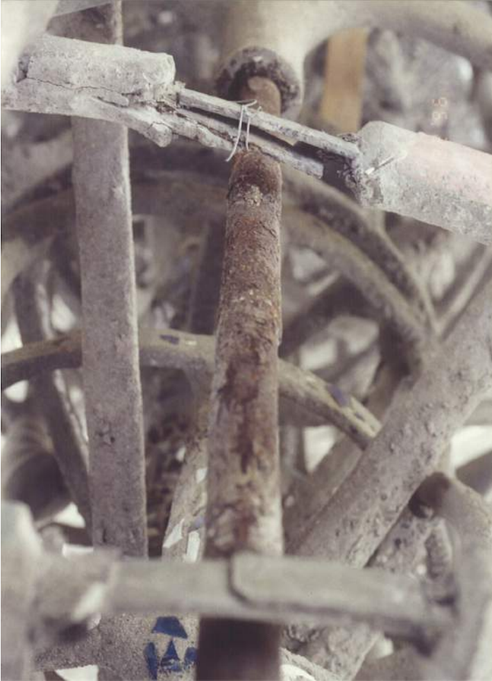
Original column and band reinforcement after opening failed coverings. May 1996
