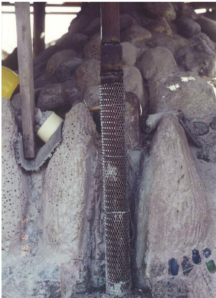
New steel reinforcement installed in Center Tower above base. Mesh has been wrapped around the pipe (left photo) and the pipe has been welded to another pipe directly above it (right photo). May 1996.
