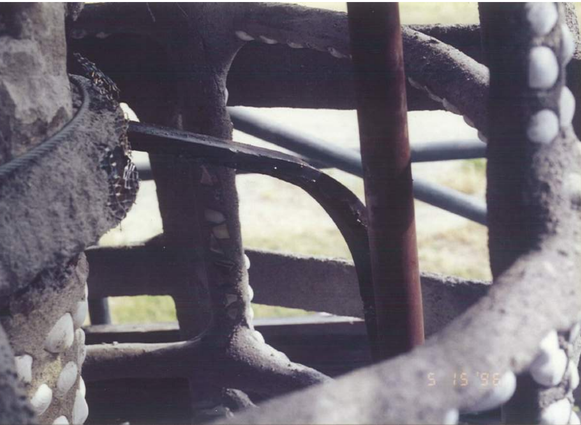
East Tower damage required repairs or replacement of reinforcements on five of six columns. At a critical junction, 19 feet above the base, the columns join the center column. The photographs depict the steel around the center column welded to the reinforcements in the vertical columns. The original Rodia covering was later restored. May 1996.
