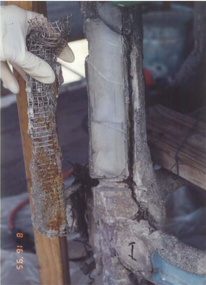
This vertical crack was the result of a major failure of a main support of the Center Tower. Bottom photo, December 1995.
