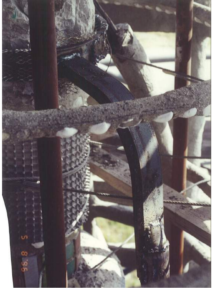
East Tower damage required repairs or replacement of reinforcements in five of six columns. At a critical junction, 19 feet above the base, the columns join the center column. The photo on the left shows a typical steel collar around the center column and the photo on the right, shows a column reinforcement welded to the collar. The original Rodia covering was later restored. May 1996.
