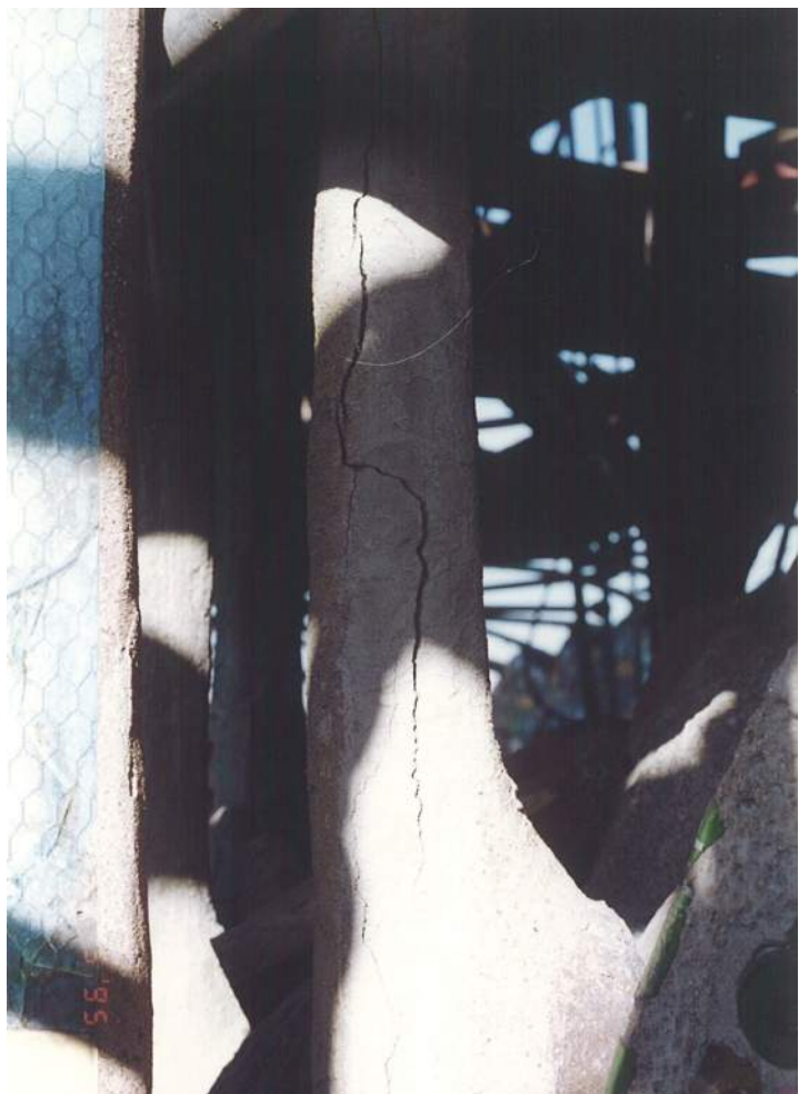
This mortar separation was found at the 74 foot level of the Center Tower. A previous repair c1981 had separated from the original mortar due to inadequate bonding. Top photo, August 1995.
