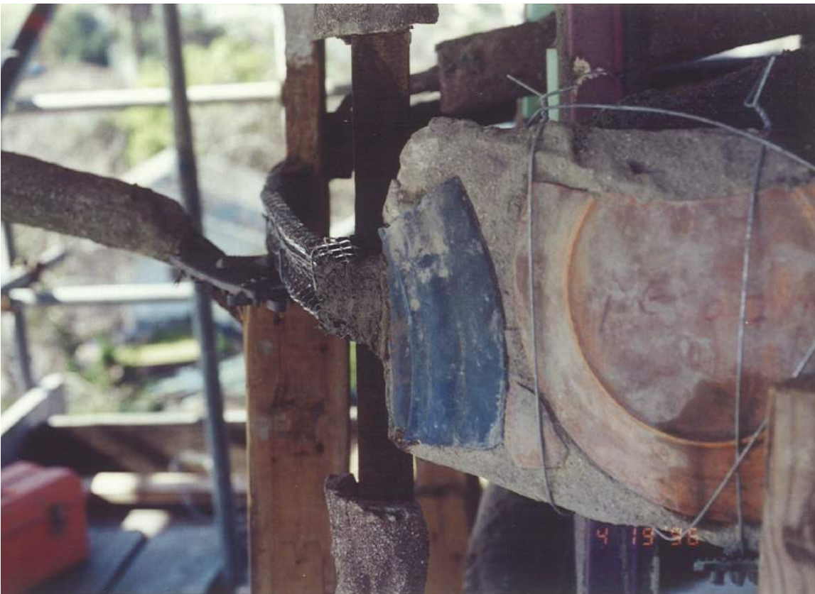
Repair in progress. Original band segments in place for installation over new reinforcement, right of photo. Major connector between Center Tower and East Tower shown at center left of photo. This connector is to be welded to column reinforcement, center of photo. April 1996.
