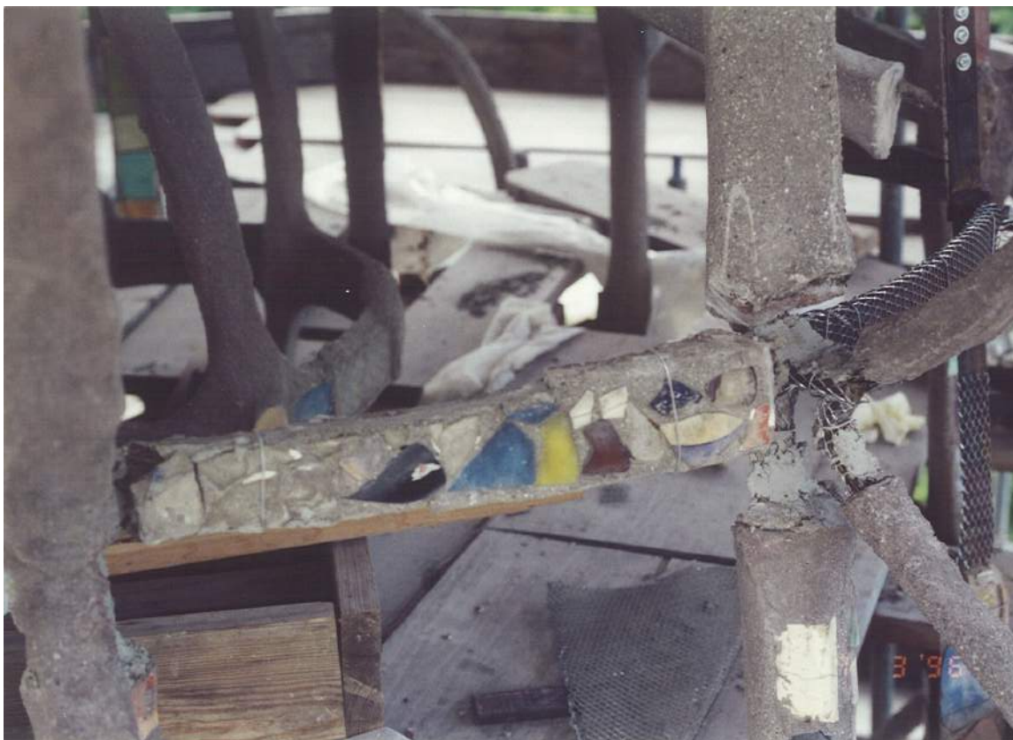
Original band covering with ornaments re-installed over repaired band reinforcement. July 1996.
