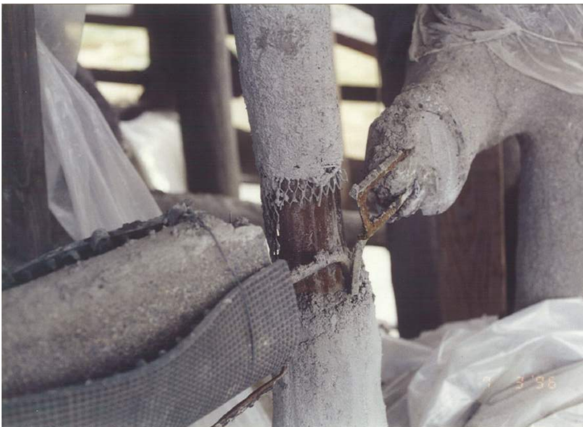
Exposed joint showing failed horizontal band reinforcement at joint with vertical column. July 1996.
