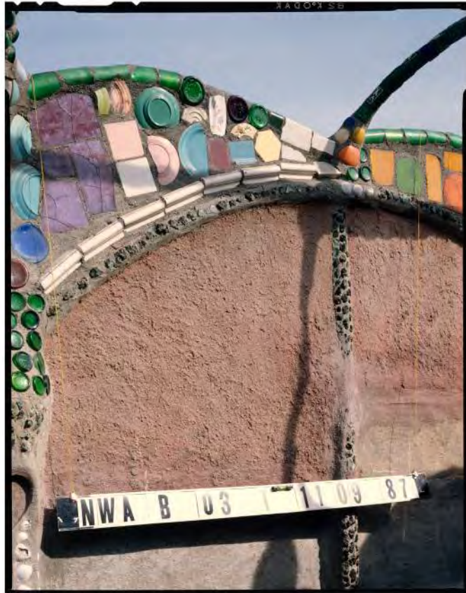
Interior North Wall Post 2 1987
