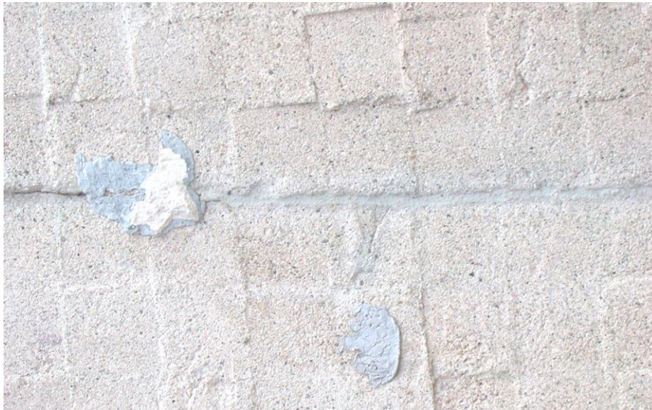
Photo 11: re-attached decoration lost (wrong adhesive)
