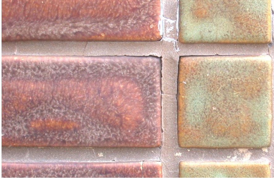
Photo 5: separation of modern re-pointing
