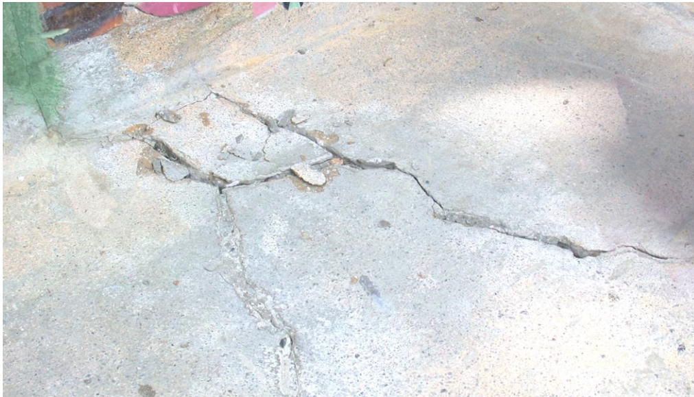
Photo 8: cracking of floor
