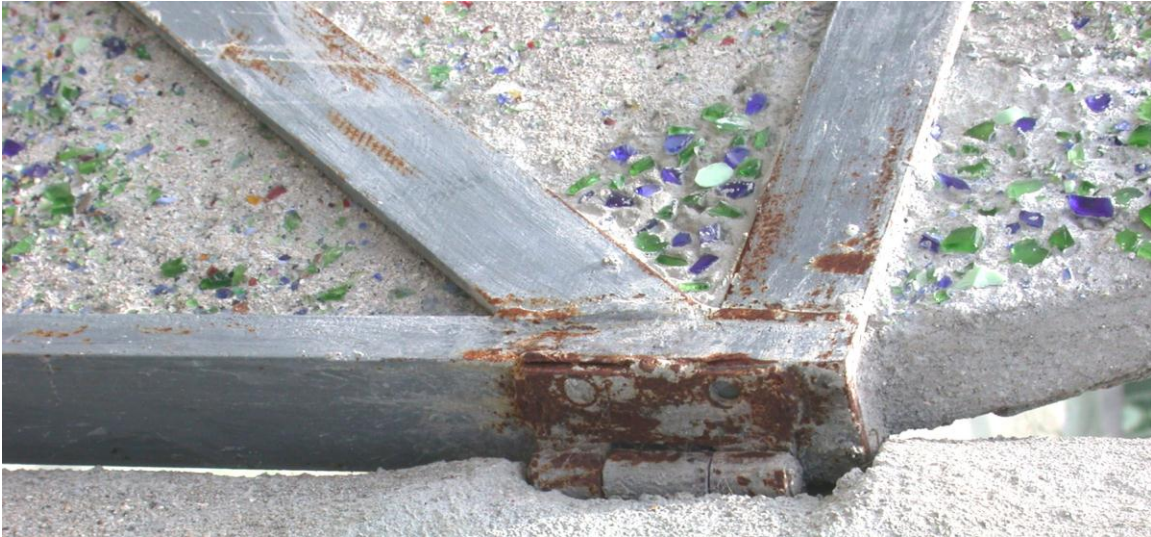
Photo 16: corroded iron door with plaster fill
