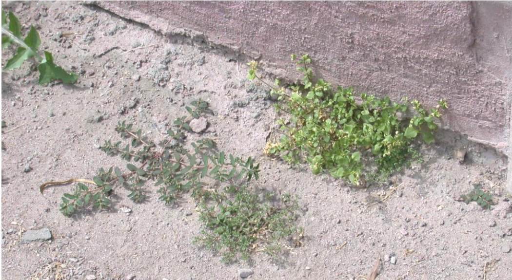
Photo 14: plants in proximity of the wall
