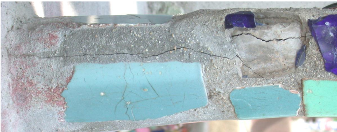
Photo 4: crack in lower elevation
