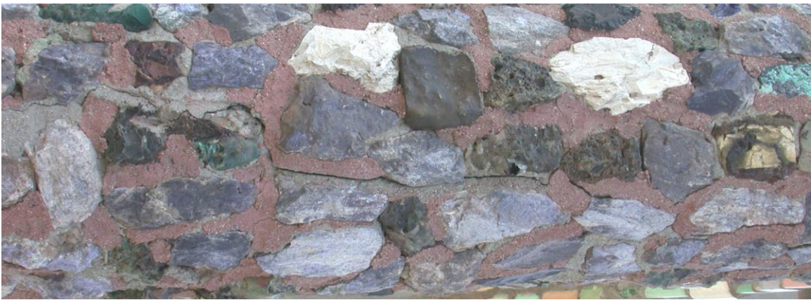
Photo 3: crack in lower elevation
