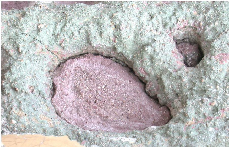
Photo 6: cracking and water access in plaster
