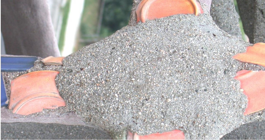
Photo 9: eroded plaster
