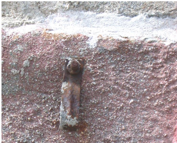
Photo 15 corroded iron anchor and mismatched patching
