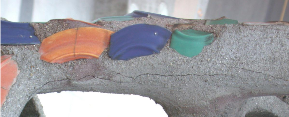
Photo 2: crack in higher elevation
