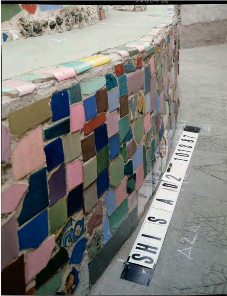
1987: Base of south side, center A and B
