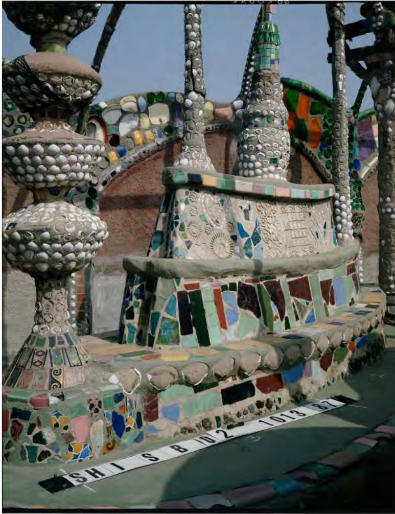
1987: South side looking northeast
