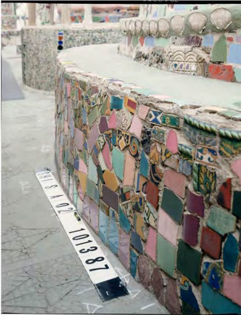
1987: Base of south side looking west, center A and B
