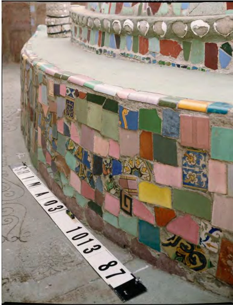
1987: Base of north side looking east, center A and B
