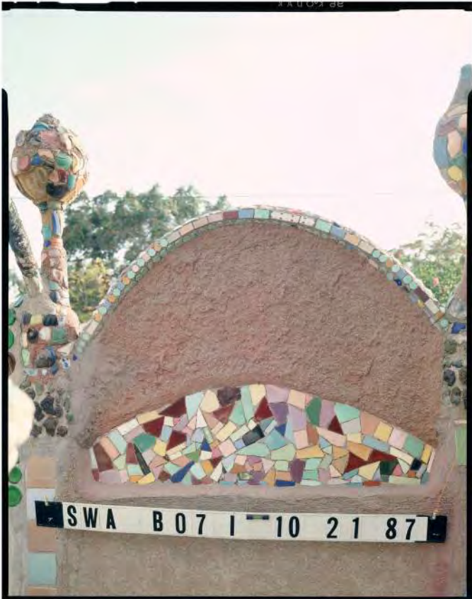
Interior South Wall Panel 7 1987
