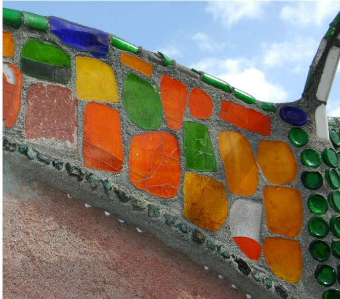
Figure 2: Interior of the North Wall, before facing.
