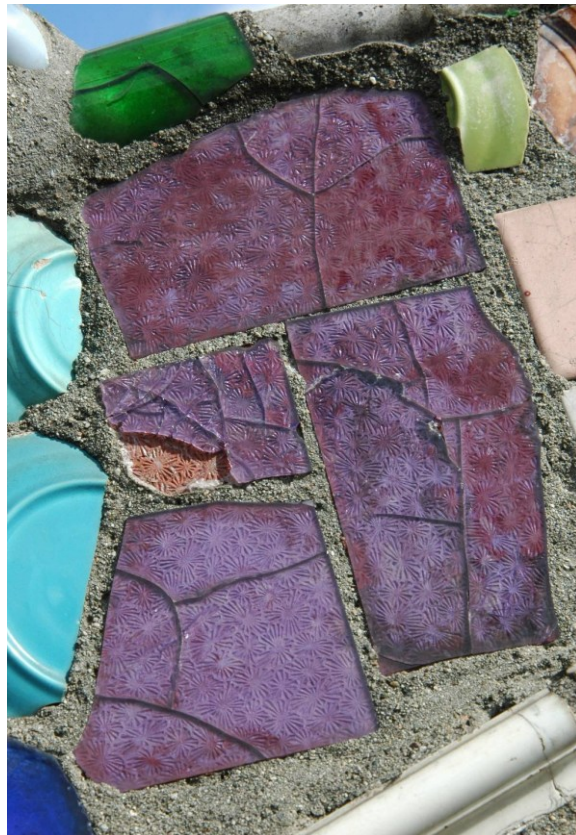
Figure 1: Detail of fractured flat glass plates on the interior of the North Wall.
