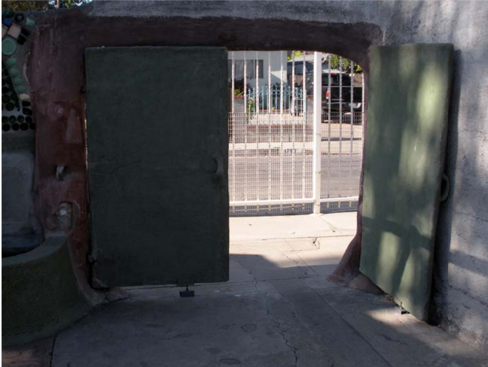
Figure 3: garage doors locked into position
