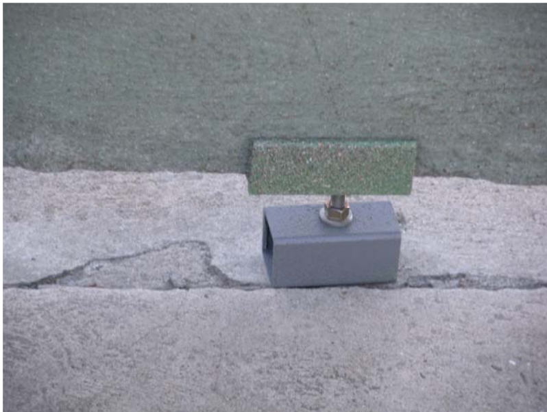
Figure 4: locking and lifting device
