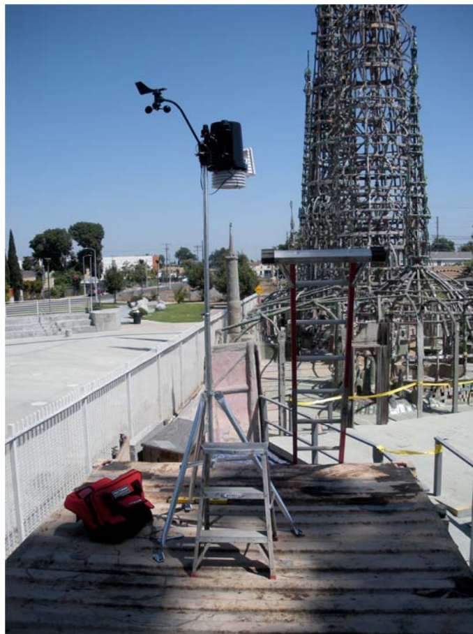
Figure 10: weather station during installation
