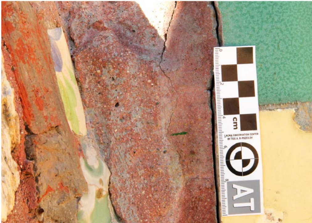
Figure 11: Crack propagation monitoring
