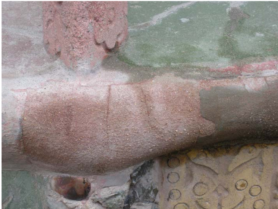
Figure 22: differential wetting of repair mortars and cracks
