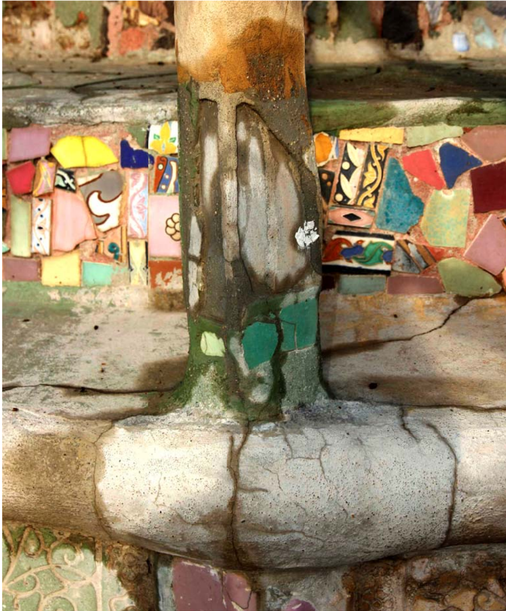
Figure 25: differential drying at WTO
