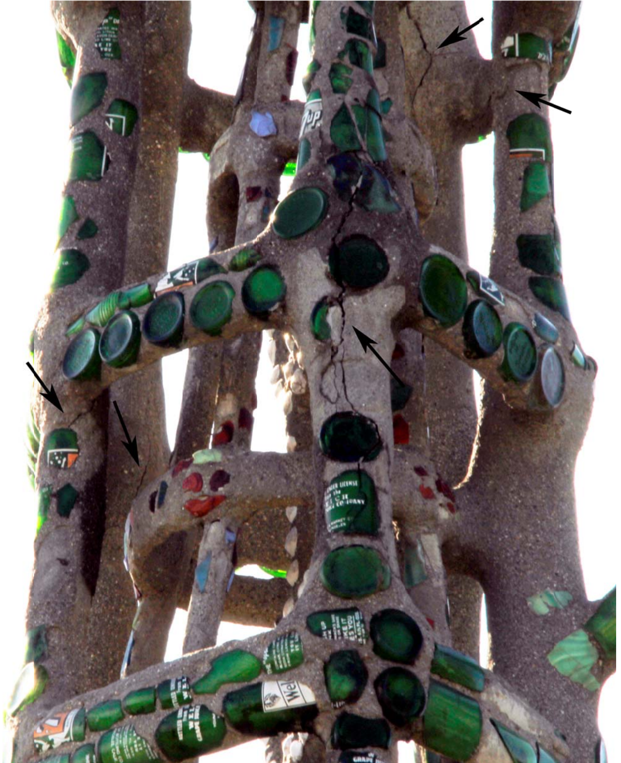
Figure 2: Detail of Top Third of the East Tower; cracks marked with arrows
