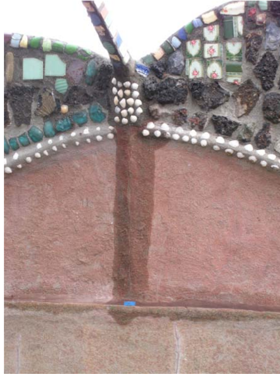
Figure 21: wetting along structural elements
