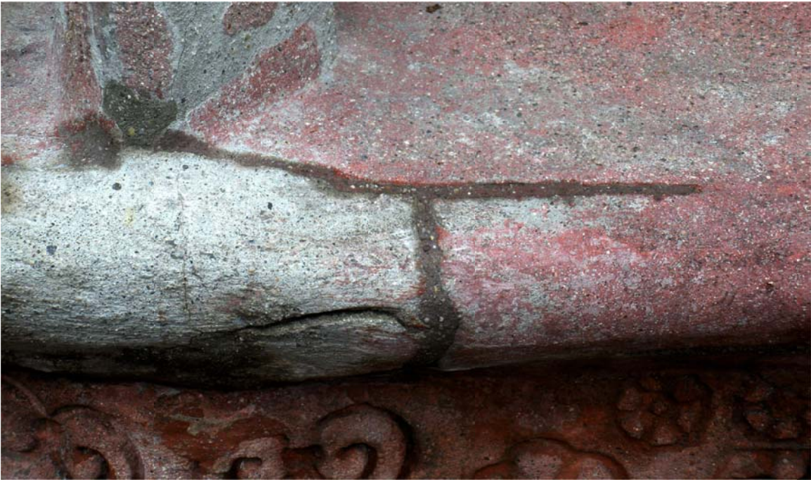
Figure 24: differential wetting of repair mortars
