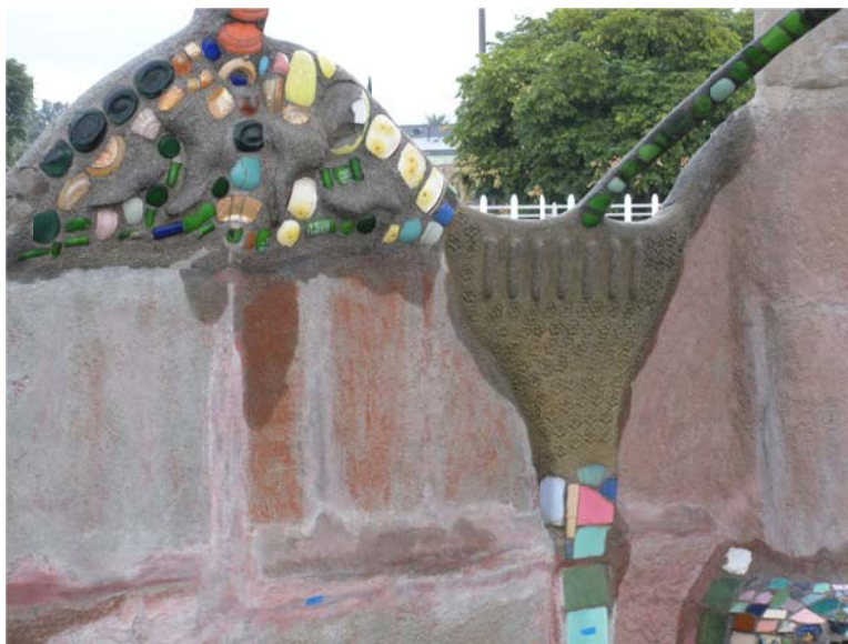
Photo 20: wetting along structural elements
