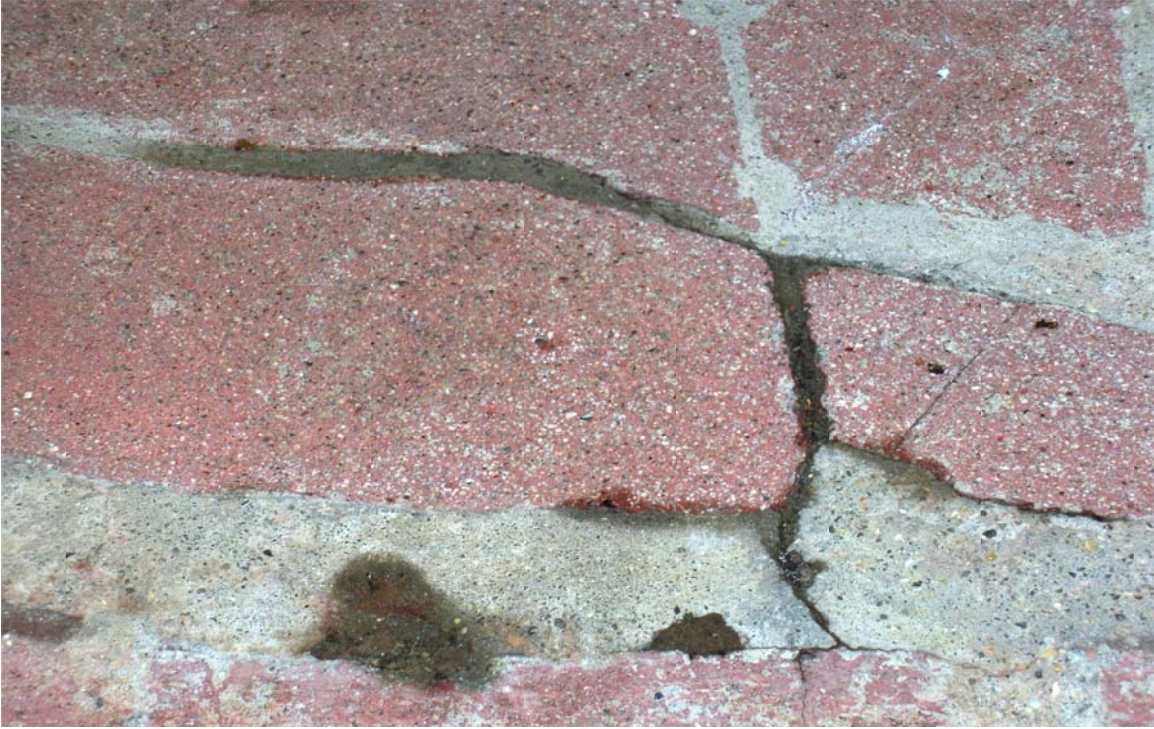
Figure 23: differential wetting of repair mortars
