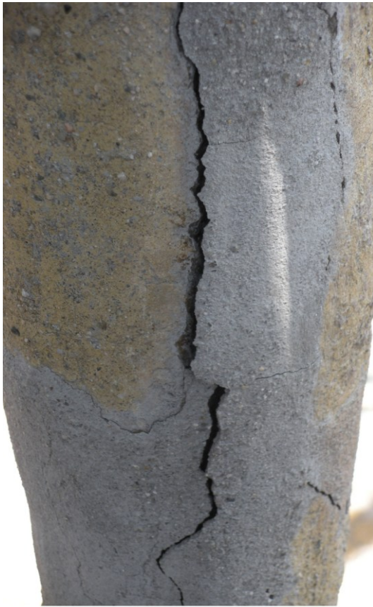
Figure 10a: failed cement mortar cover
