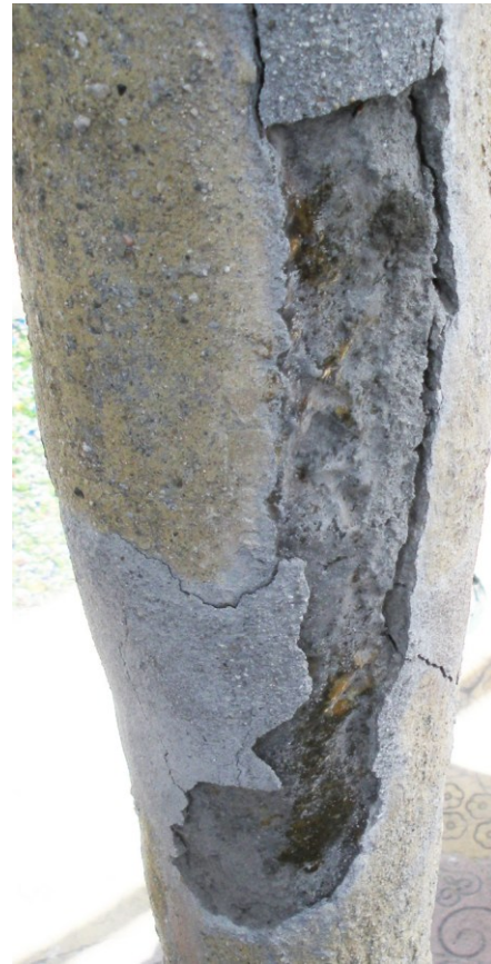
Figure 10b: exposed epoxy mortar after removal of failed cement mortar cover
